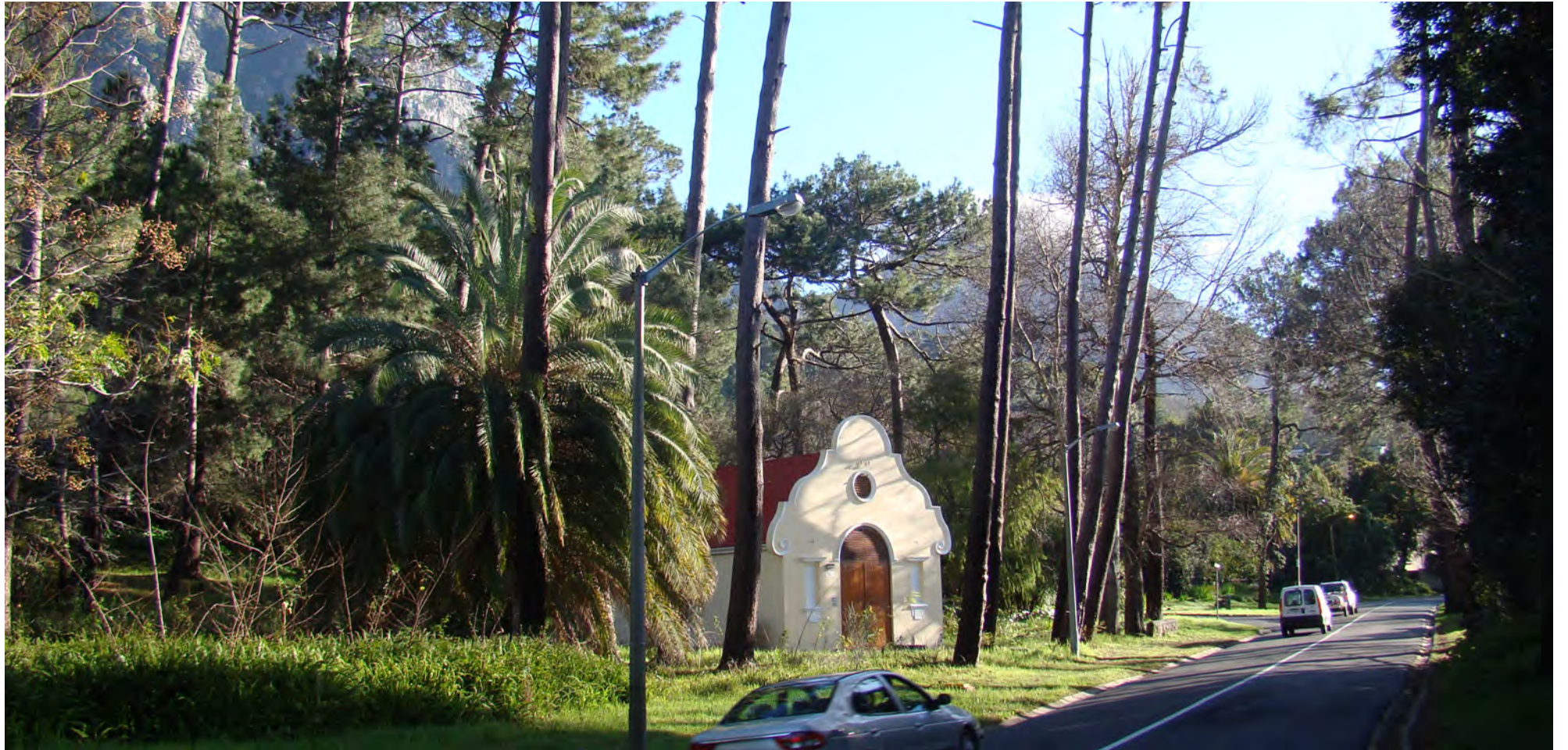
Figure 2.6- The site, taken from Rhoads Drive, the substation presents itself as a monument
