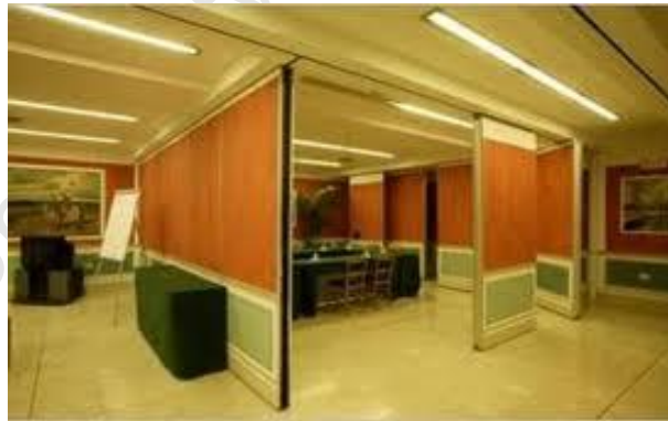
Figure 2.13: Aluminium partition (Newbury Interiors, 2007)
