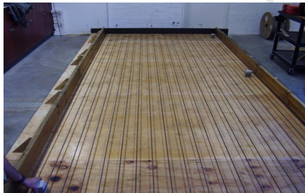
Figure 5.2: Formwork before concreting
