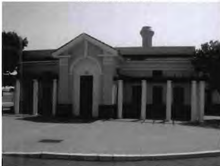
50: GREENPOINT PUMP STATION
