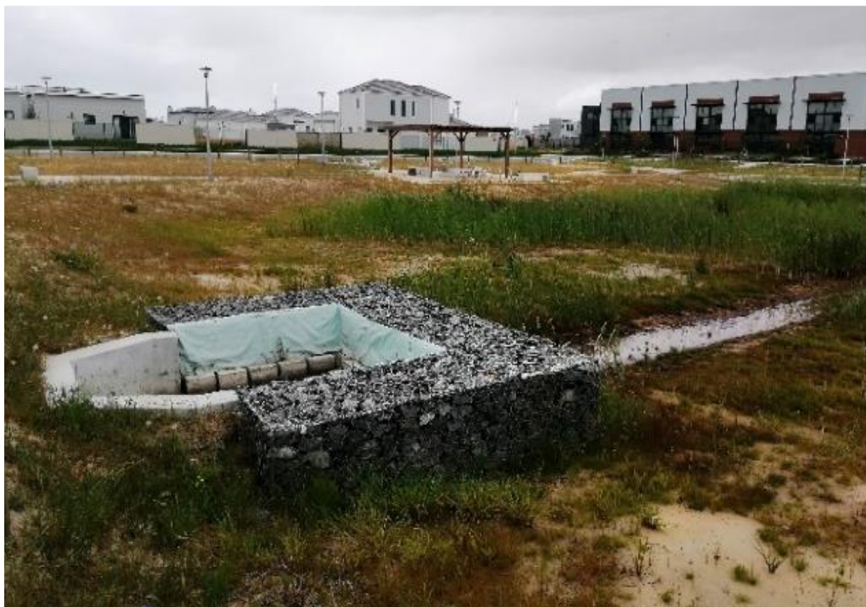
Figure 2-6: Forebays at a development in Parklands, Cape Town, South Africa
