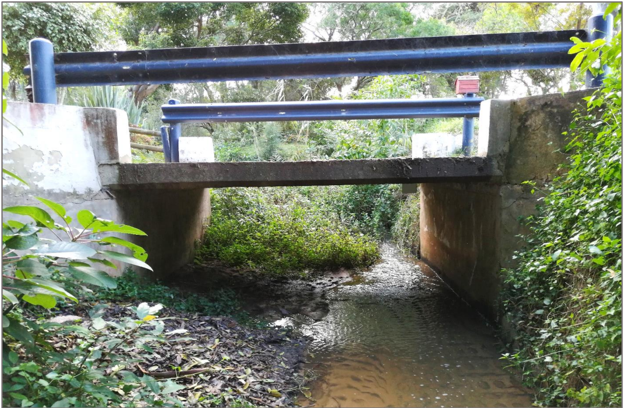
Figure 5-5: Old Place Stream Sensor (Bo 7) beneath a private bridge
