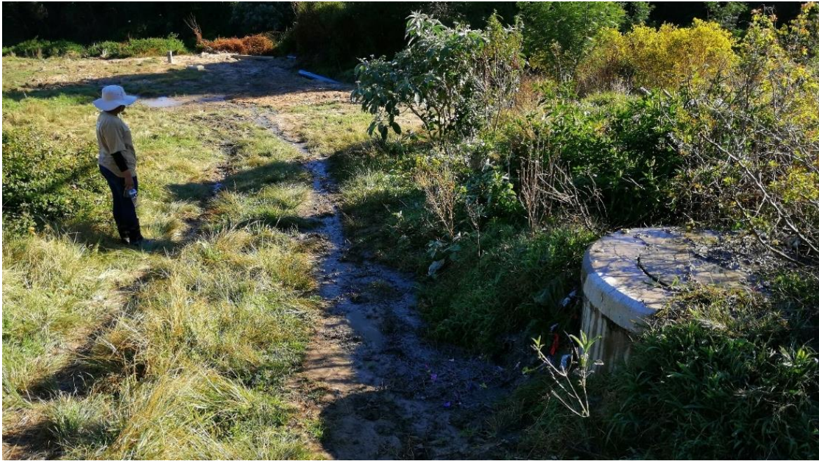
Figure 8-2: A manhole sewage overflow problem at a gradient transition
