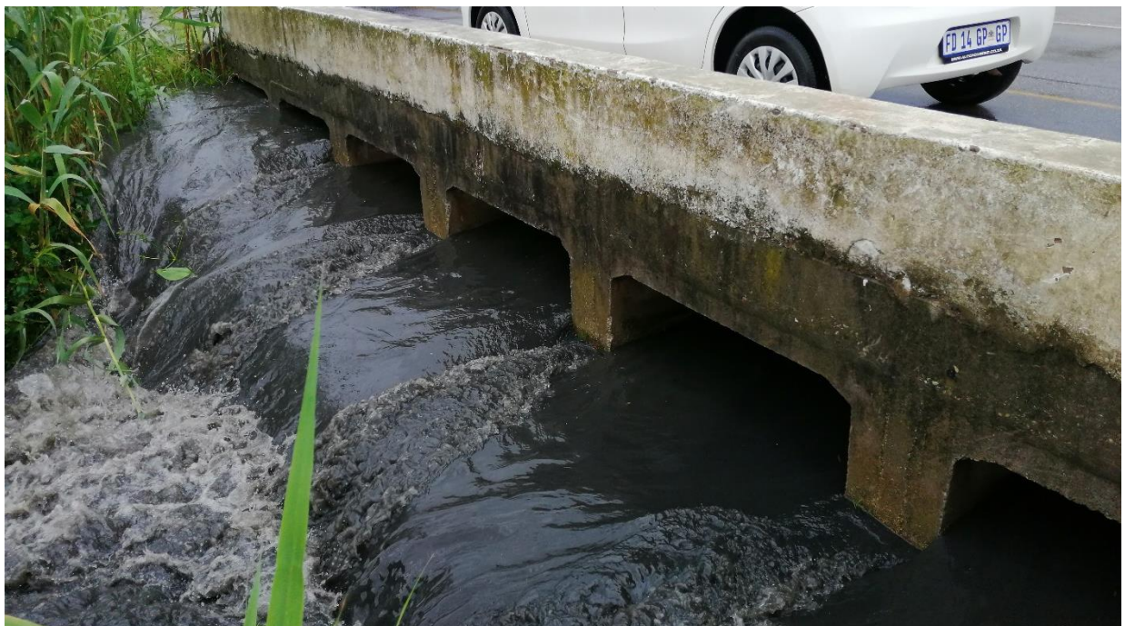
Figure 3-19: The outflow of the Bongani River wetland beneath George Rex Drive
