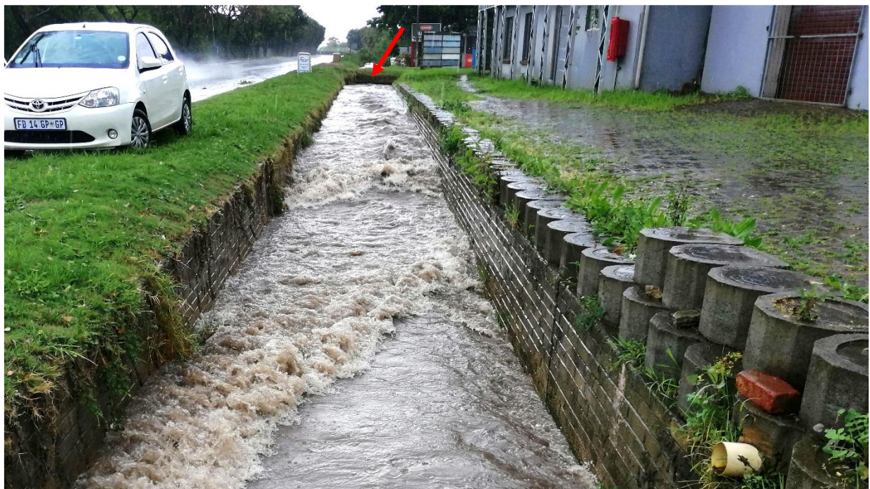
Figure 5-4: Vigilance Canal Sensor location (Bo 12) beneath Sandpiper Street Culvert
