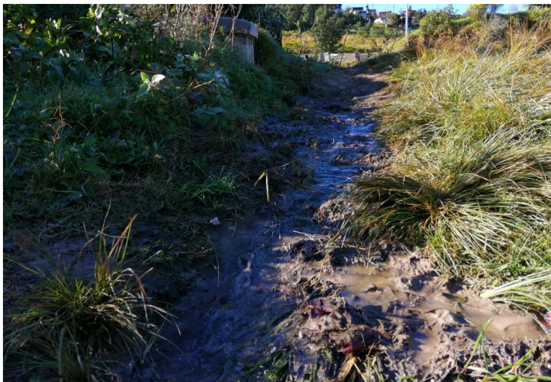
Figure 8-11: Sewage overflow from a manhole at a change in gradient in the sewerage, flowing overland towards the Bongani River
