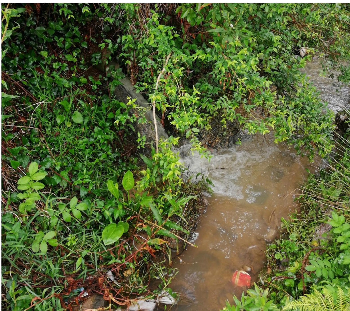
Figure 7-11: Bongani 2A sample site showing the sewage overflow into the stream
