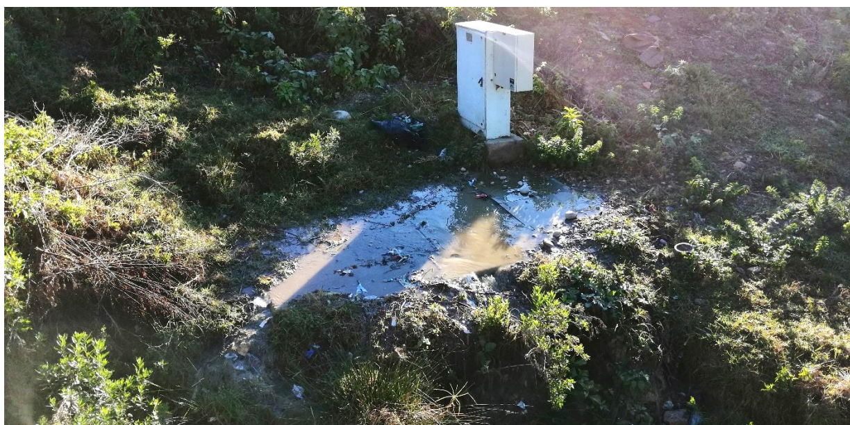
Figure 8-10: Point source pollution from an overflowing manhole in Joodse Kamp
