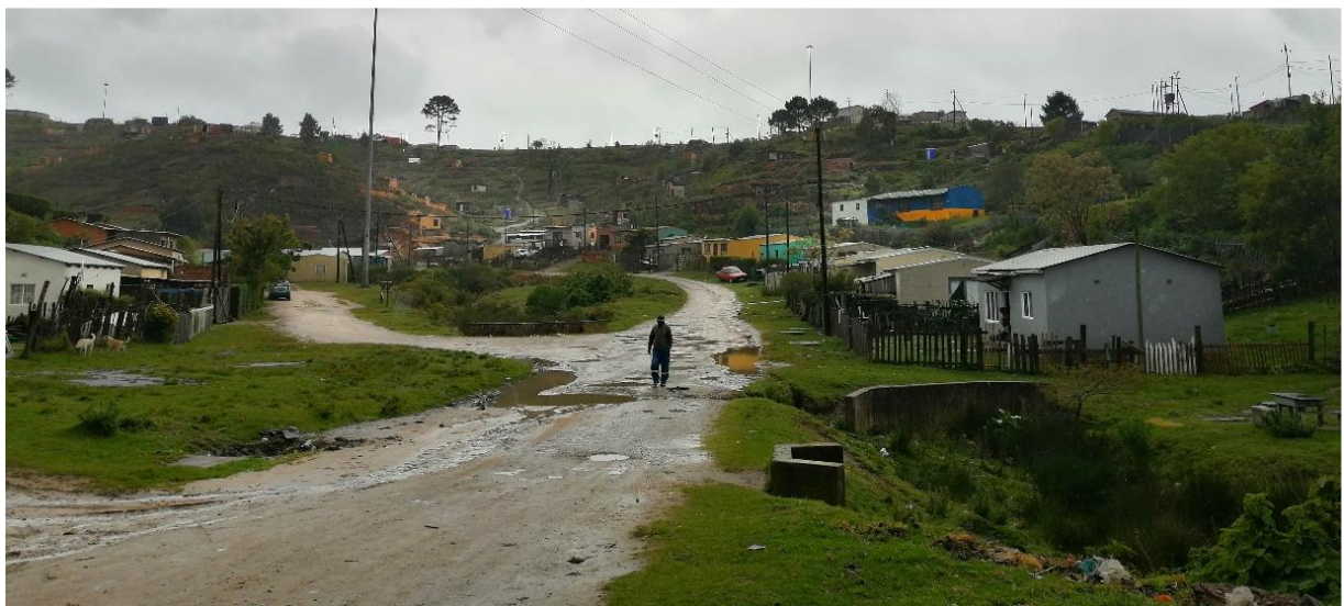
Figure 8-8: The poor drainage of the low-income settlement of Bongani
