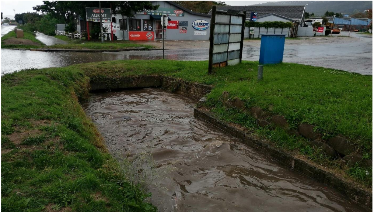
Figure 3-18: Vigilance Canal flowing beneath Sandpiper Street
