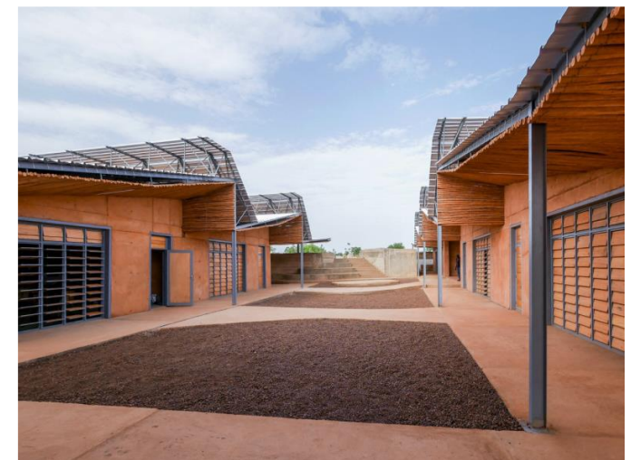
FIGURE 35: Burkina Institute of Technology Looking into Courtyard Space
