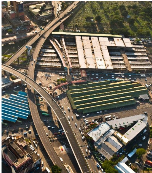
FIGURE 42: Aerial View of Warwick Junction Around Different Transport Nodes
