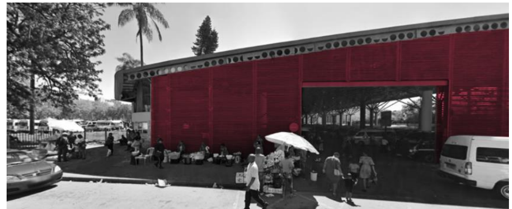
FIGURE 81: Market Taxi Rank Highlighting the Metal Shell Proposed to be Removed from the Structure
