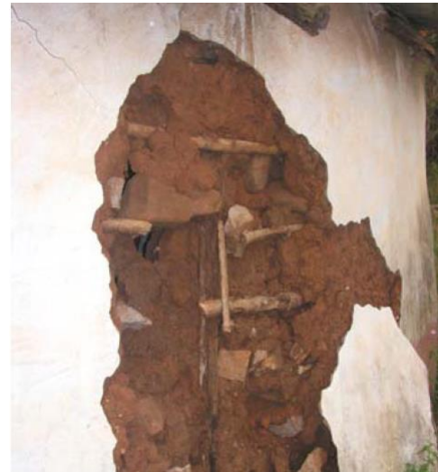
FIGURE 30: Earth Walls Being Used as Infill to Enclose Frame Structure
