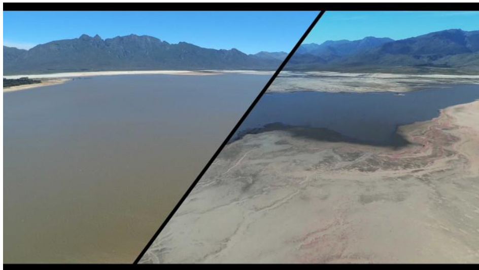
Figure 1.6 Before and after photos of the Theewaterskloof Dam following the 2016 drought.
