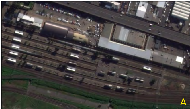
Figure 5.1 Bellville rail station platforms
