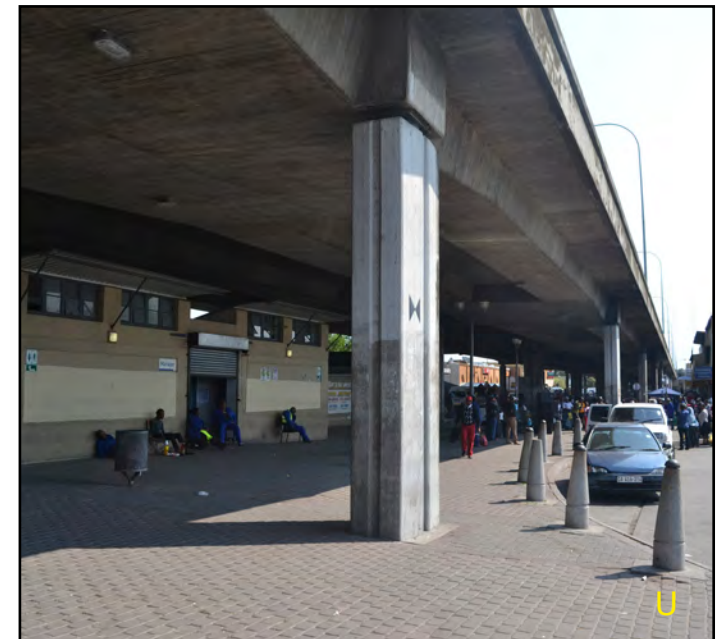
Figure 5.35 Poor lighting and safety under the Tienie Meyer Bypass
