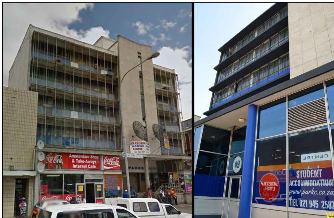
Figure 5.36 Transformation of building from commercial use to student housing
