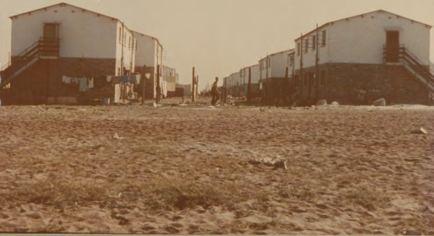
Site after construction, 1971.
