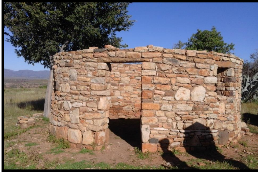
Figure 4.21: Queen 'Mamohato's newly restored hut.
