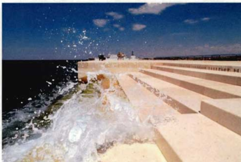
fig 85 These steps were designed by Nikola Basic to play specific notes through pipes much like an organ. Located on the quayside of Zadar, Croatia, there are 35 musically tuned tubes with whistle openings on the sidewalk - depending on the size and velocity of the wave - musical chords are played.
