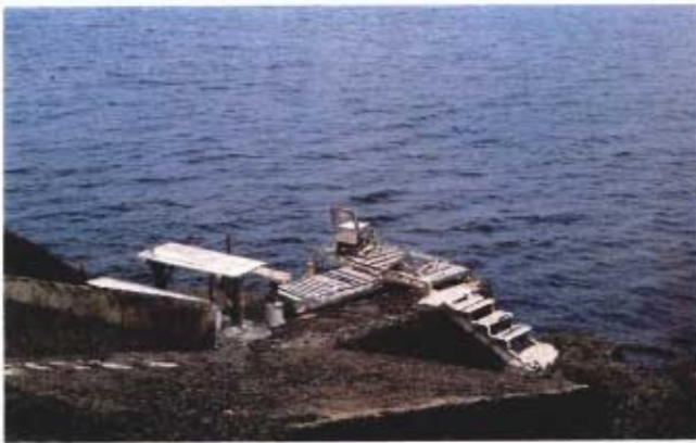
fig 79 Fishing pitches in the port of Barcelona, Spain (Daidalos, 1997. Topographic Extremes. Vol. 63)
