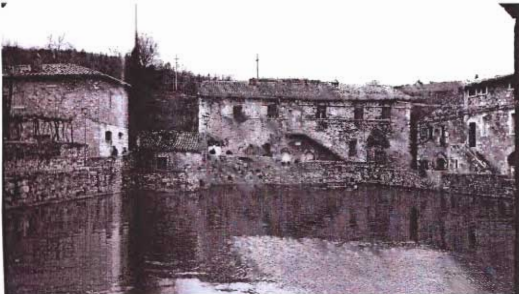
fig 43 The basin of Bagno Vignoni in Southern Tuscany (Daidalos, 1995, Aquatic Arts, Vol. 55) The springs of the small Tuscan city were already used as thermal spas by the Romans. The regularised basin is chisled out of the bedrock.
