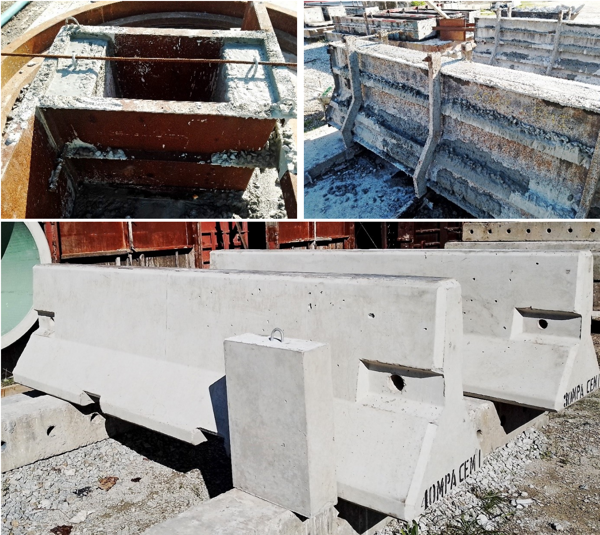
Figure 3-5 Cast median barriers and 'mock panel' (bottom), placed concrete in steel formwork, panels (top-left), and barriers (top-right).
