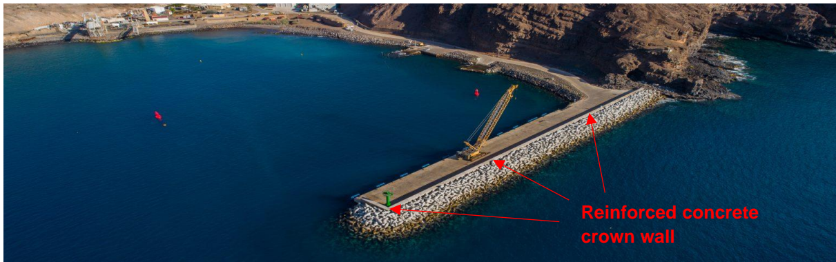
Figure 4-5: An aerial photograph of the completed breakwater in Rupert's Bay, St. Helena Island (PRDW, n.d.).
