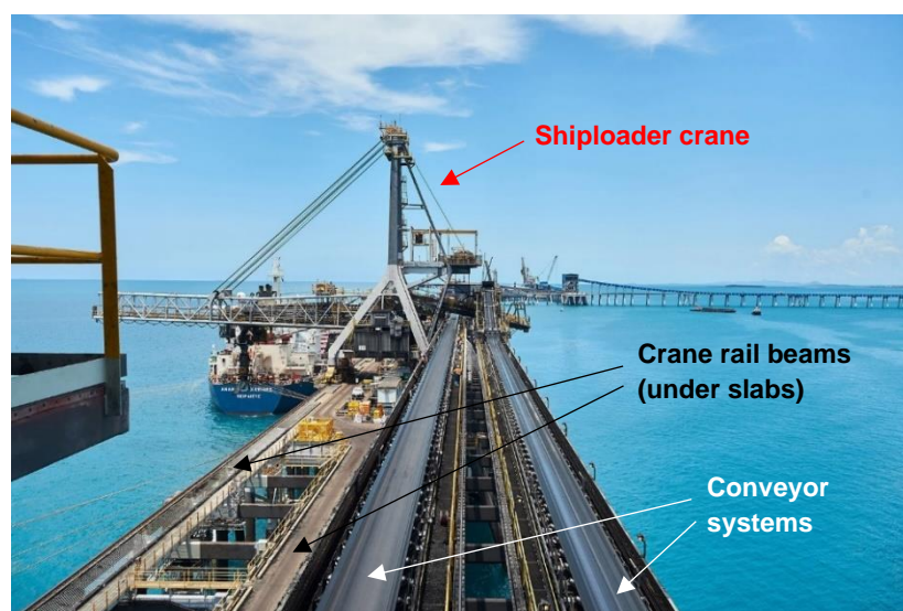
Figure 4-1: A typical RC coal export jetty in Dalrymple Bay, Australia (adapted from Dalrymple Bay Coal Terminal, n.d.). Note the shiploader crane, conveyor systems, and crane rail beams.
