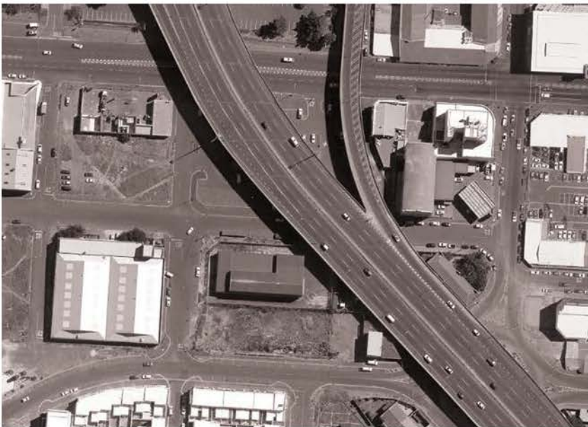
Fig.4 Aerial view of District Six Bypass Google Maps (2017)
