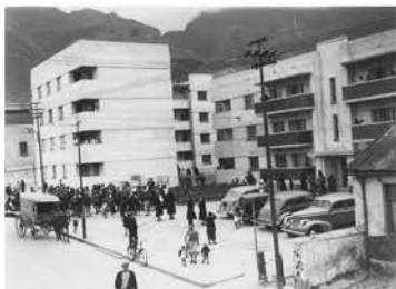
Bloemhoff flats built in the 1930s after slum clearance of Wells Square
