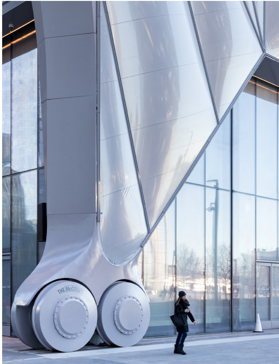
FIGURE 111 : Exterior of 'The Shed' showing ETFE Cushion facade system, structure and 'bogie wheels'. Photo by Iwan Baan (2019)
