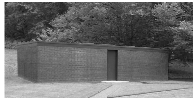
FIGURES 31 AND 32 : Exterior and interior views of 'The Guest House'
