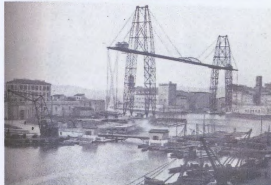
Harbor of Marseilles. (Sigfried Giedion, Bauen in Frankreich ) Giedion comments: "A mobile ferry suspended by cables from the footbridge high above the water connects traffic on the two sides of the harbour. This structure is not to be taken as a 'machine'. It cannot be excluded from the urban image, whose fantastic crowning it denotes. But its interplay with the city is neither 'spatial' nor 'plastic'. It engenders floating relations and interpretations. The boundaries of architecture are blurred."
