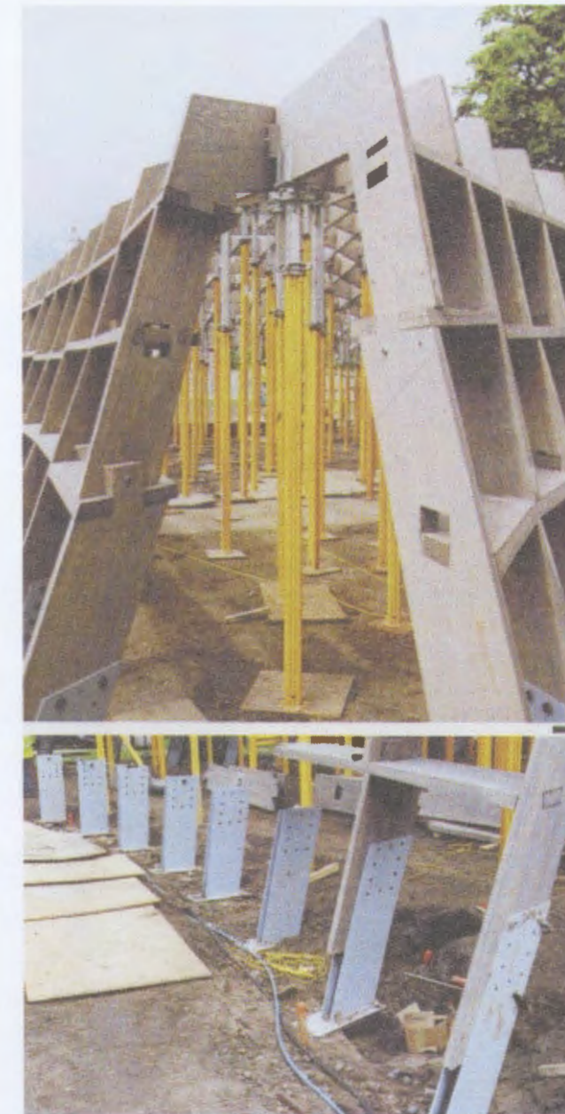
assembly process showing steel shoes and over lapping joints.
