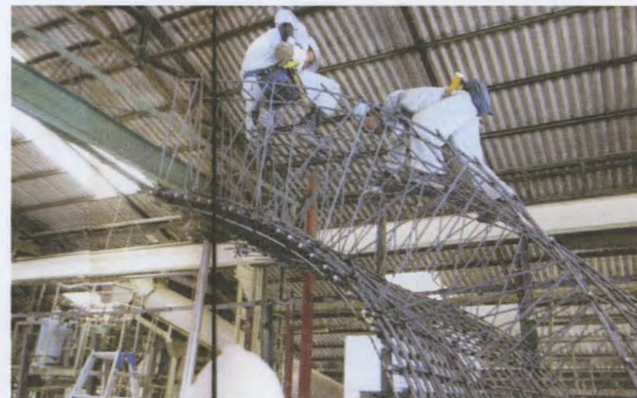
Prototype of the proposed Catenoid structure being assembled in a factory
