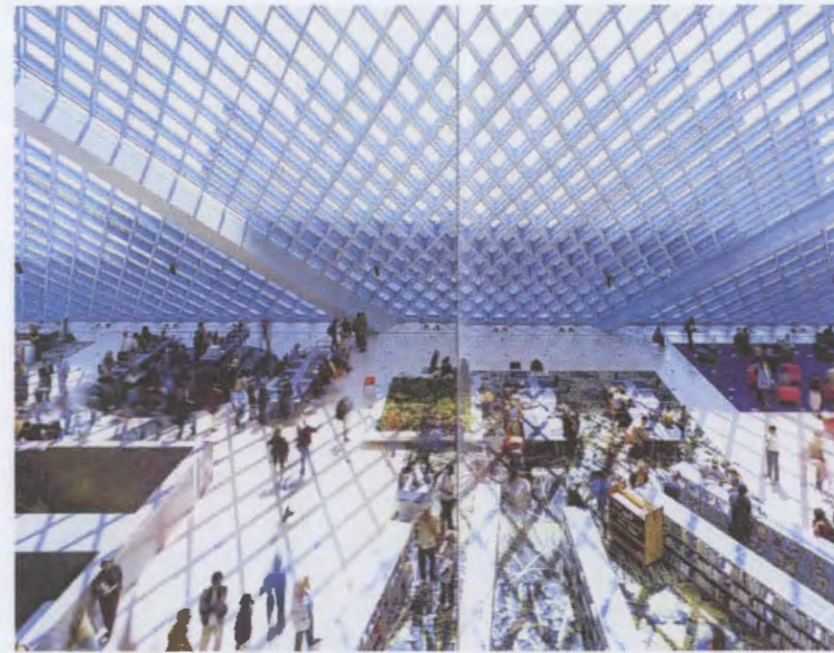
Interior view showing slanted diamond-grid-skin
