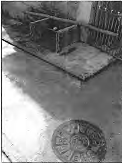
Fig. 5.9 Sete de Setembro, Sao Paulo: An edge has been added to this 1.4m-wide pedestrian pathway to increase its stormwater carrying capacity, while waterborne sewers run down the centre. Note the right-angle bend in the path to fit between existing dwellings.
