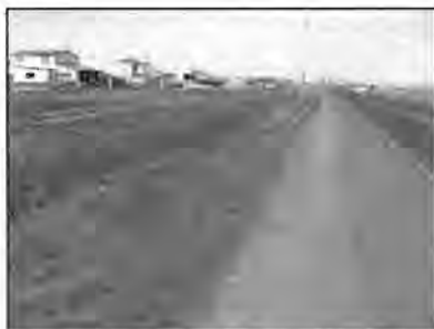
Fig. 4.13 A filter strip on a road verge
