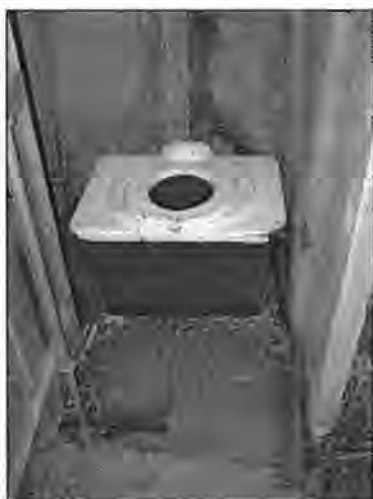
Fig. 2.12 A bucket toilet typical of those supplied to informal settlements in the Western Cape
