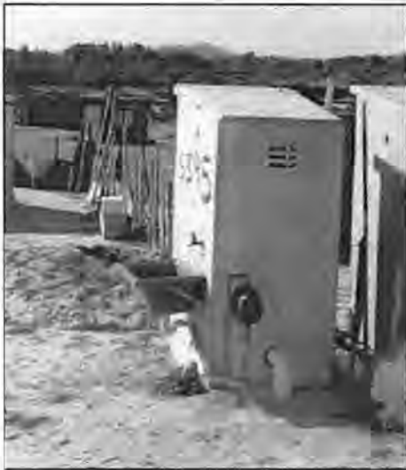
Fig. 3.3 A yard connection attached to a sewerage toilet block in a 'sites-and-services' type development
