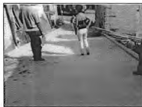
Fig. 4.11 A cast in-situ dished road surface
