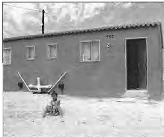
Fig. 3.2 An 'RDP' house with metered, in-house water supply and water-borne sewerage
