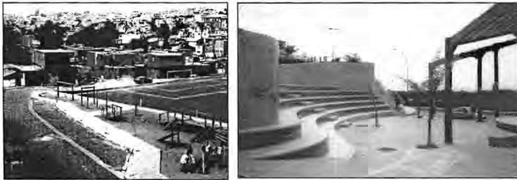
Figs. 5.11 and 5.12 Upgraded settlements in Sao Paulo and Rio de Janeiro, Brazil, where hardened spaces were provided as recreation areas with playing equipment, benches, steps and vegetation. In many projects the recreational areas were created before any of the infrastructure was provided to prevent invasion of the open land (Source: M Carrilho Arquitos, 2000:206 and N Graham).
