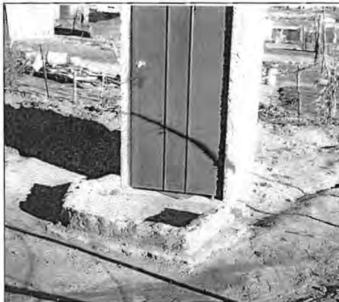
Fig. 4.6 A concrete bund built by the user of a composting toilet in Elias Motsoaledi township, Johannesburg, in order to keep out stormwater (Source: Stewart Scott, 1998:11)
