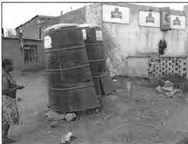
Fig. 2.11 A chemical toilet in Kliptown, Gauteng (Source: DWAF, 1999)
