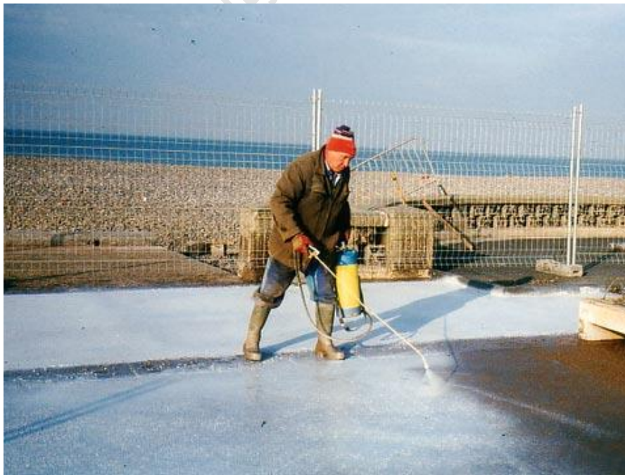
Figure 14: Application of Membrane-Forming Curing Compound ( http://www.planete-tp.com/en/concrete-curing-a249.html )
