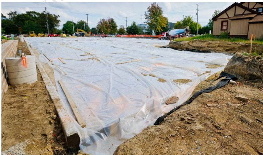
Figure 11: Plastic sheeting acts as an effective sealing method
