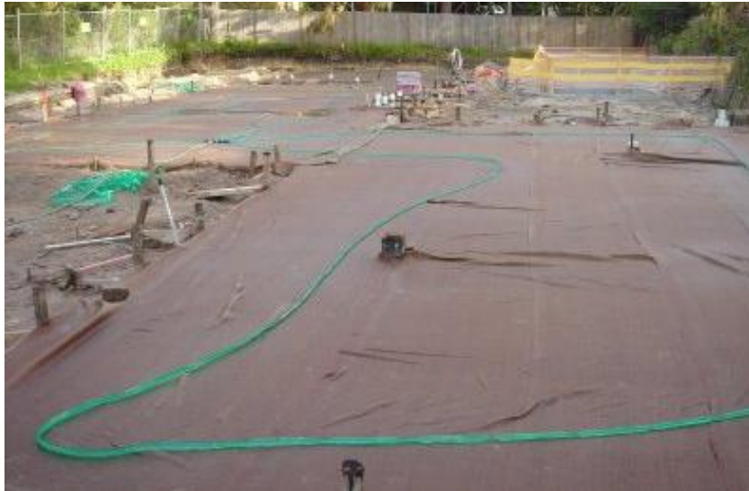
Figure 8: Hessian cured concrete slab
