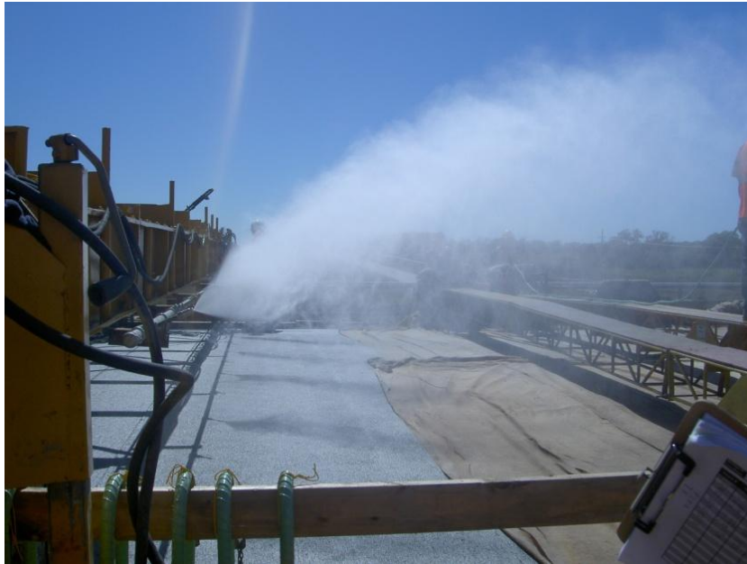
Figure 6: Fogging of newly placed concrete
