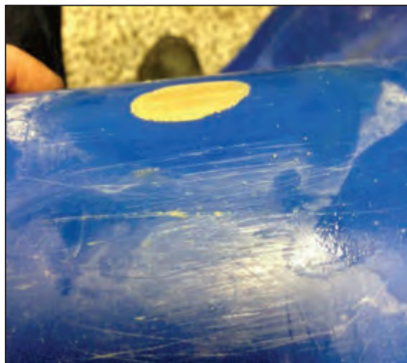
Figure 3-14: Putty Taking on the Original Pipe Profile
