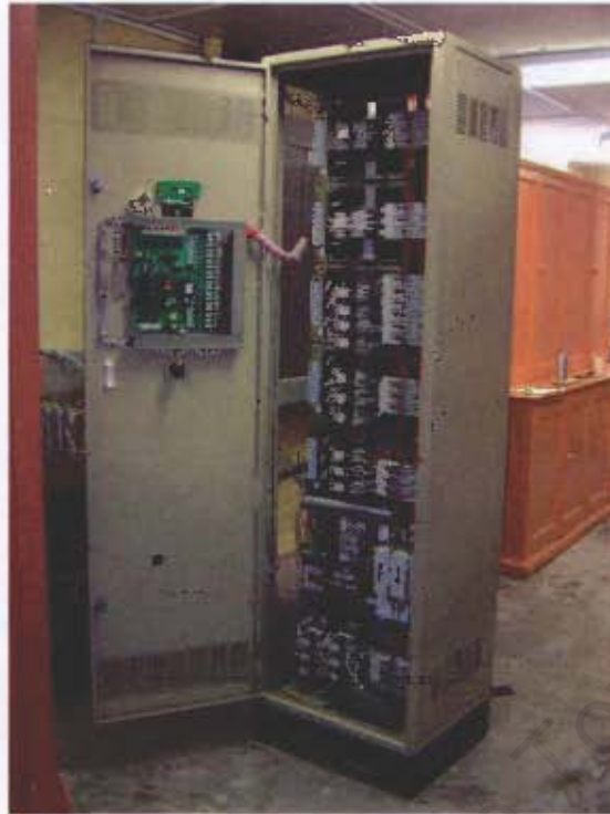
Figure 71: Photo - Completed Installation
