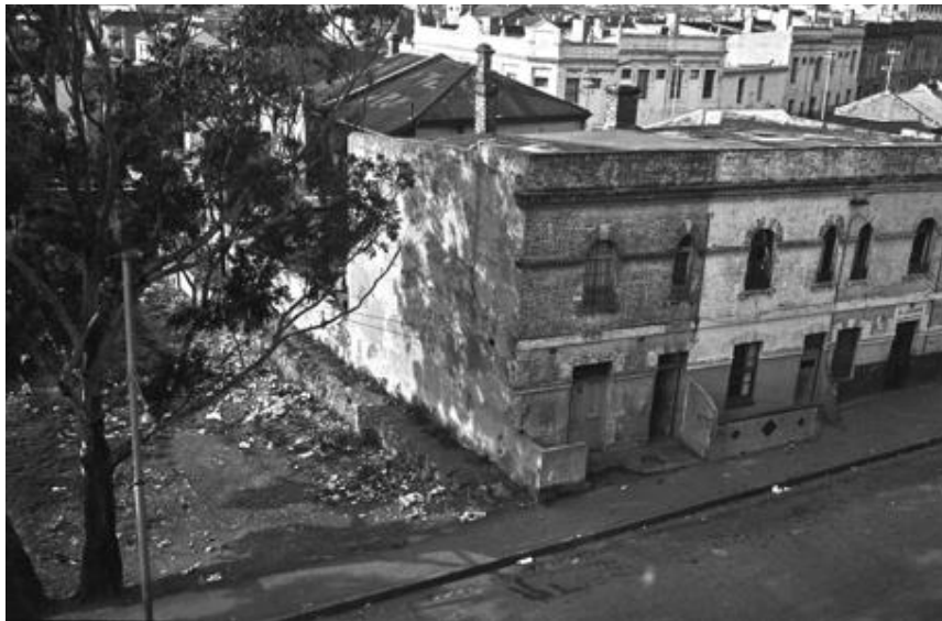
Figure 7: Mid-19th century back-to-back housing in District Six. The photograph shows dense urban residential development fronting onto the street and few opportunities for air and ventilation. Conditions were exacerbated by overcrowding. There is evidence of a small lane to the left of the photograph. The area is in the process of demolition. (City of Cape Town CCb134_56_s4-i16)
