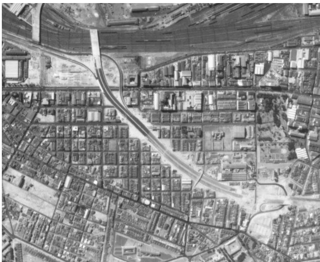
Figure 91: This aerial photograph dated 1968 shows the Eastern Boulevard, now completed, cutting through District Six. Some 240 houses were demolished to make way for it. (Photograph: CoCT)
