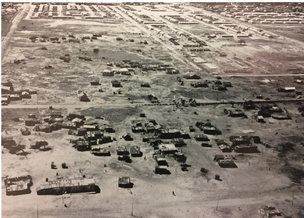
Figure 79: Re-ordering city spaces in action: Windermere in the process of demolition, giving way to the planned township of Factreton. Windermere was an ongoing target of slum clearance, from its inclusion in the municipal area in 1946 until the completion of Factreton and Kensington, in addition to raids and forced removals throughout the 1950s. (City Engineer's Report 1960, CoCT)
