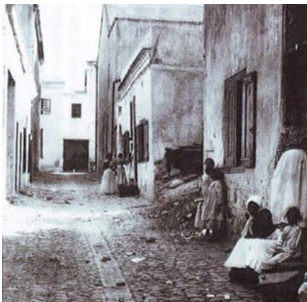
Figure 4: Huurhuise in Coffee Lane, Cape Town, since demolished. This early housing type was constructed in the mid- to late-18th century within the narrow lanes of Cape Town which interspersed the historic city blocks. An early huurhuis would have had no water provision or waterborne sewerage. There were waste traps that were filled with detritus which would be cleared occasionally with sea water. Conditions were made worse by overcrowding (Elliot Collection KAB.E7979)
