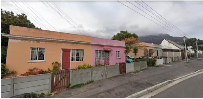
Figure 35: Houses in Jutland Avenue, Vredehoek, are the remaining examples of the Roeland Street Housing Scheme for council workers. Most of the verandas in the plan above have been filled in for extra space. (Photograph, 2023)
