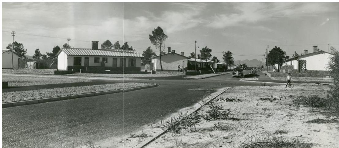
Figure 61: Early suburban houses on the Cape Flats, Kewtown, c1940. These houses were developed according to a standard CTCC typology and were generally semi-detached. Houses were placed at angles to one another for variety and improved ventilation, a reaction to the tight inner-city housing they replaced, and some were arranged around a 'woonerf' concept which excluded cars and favoured pedestrian use. These houses were generally more spacious than those that followed. (ANA va_independent_S5C_029)
