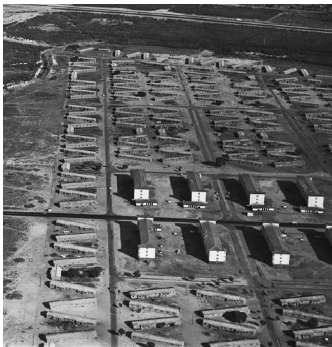
Figure 65: The Old Flats at Langa built after 1944. They comprised eight four-storey blocks with rooms housing two men per room. The cottage-style hostel blocks were called 'the Zones'. (CoCT CCb122_f17_i04)
