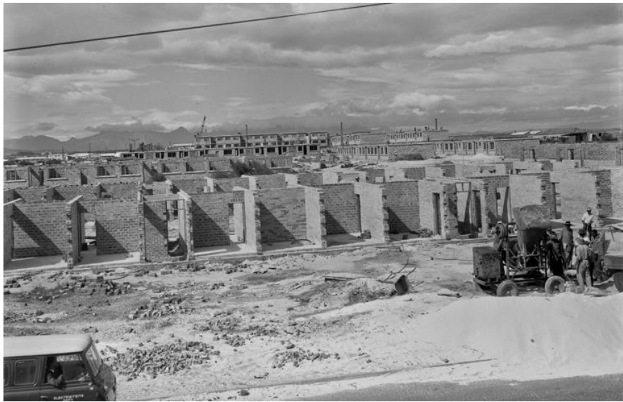
Figure 103: Modern mass-construction methods: site not identified but probably Gugulethu. (CCb130_f46_i03)
