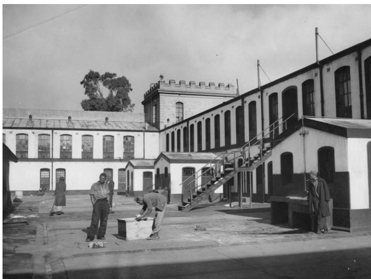
Figure 45: Docks Location at the old Breakwater Prison, now the UCT Graduate School of Business. The Docks Location moved to this facility after the original corrugated iron barracks were dismantled by 1930. The central courtyard is the controlled area within which all communal activities would take place. There was a single entrance where access could be monitored. (No date, va_independent-S8F_025)
