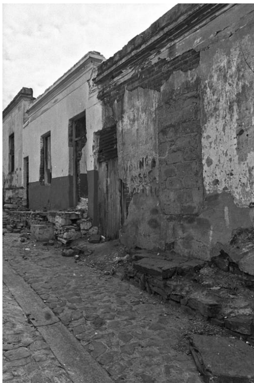
Figure 49: An abandoned row of houses in District Six ready for demolition c 1970. Although no longer inhabited, it shows the structural issues of tight inner-city living that modern town planners objected to – the narrow lanes, the housing and balconies spilling onto the street and the central stormwater drainage system which used to collect detritus. (CCb132_f40_s5_i127)
