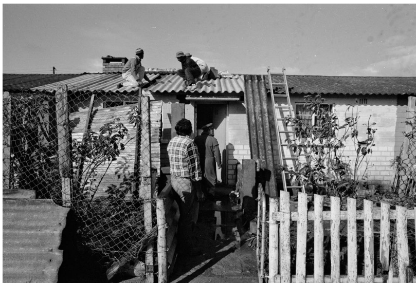
Figure 93: Fixing the roof of a typical mass-produced NE 51/10 house. Site not identified. Roofs were corrugated asbestos, although most houses eventually had ceilings. Plan for the row house type (CoCT). The NE 51 typologies facilitated mass housing for the working classes. However, the results altered the shape and form of Cape Town as a city, creating the large-scale segregation of residential spaces which formed the basis of an apartheid city. (Photo c 1955: CCB176_f74_s2_i6)
