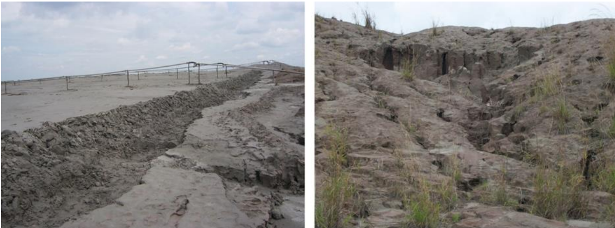
Figure 11: Erosion on the old dry tailings. Pictures courtesy of Lewis Tumbama, 2008
