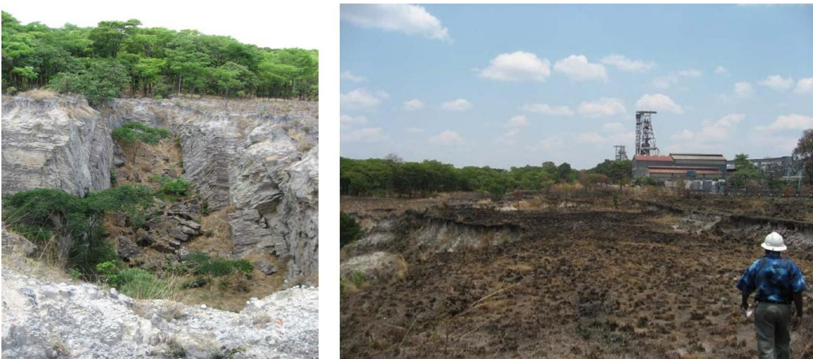
Figure 12: Land subsidence and caving above the underground workings in Luanshya. Source; Luanshya Copper Mines, decommissioning and closure report, 2007. Annexure 3.
