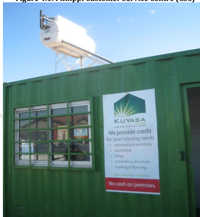
The CSCs have solar energy on display as seen with the solar water heater on top of the container. Source: Author
