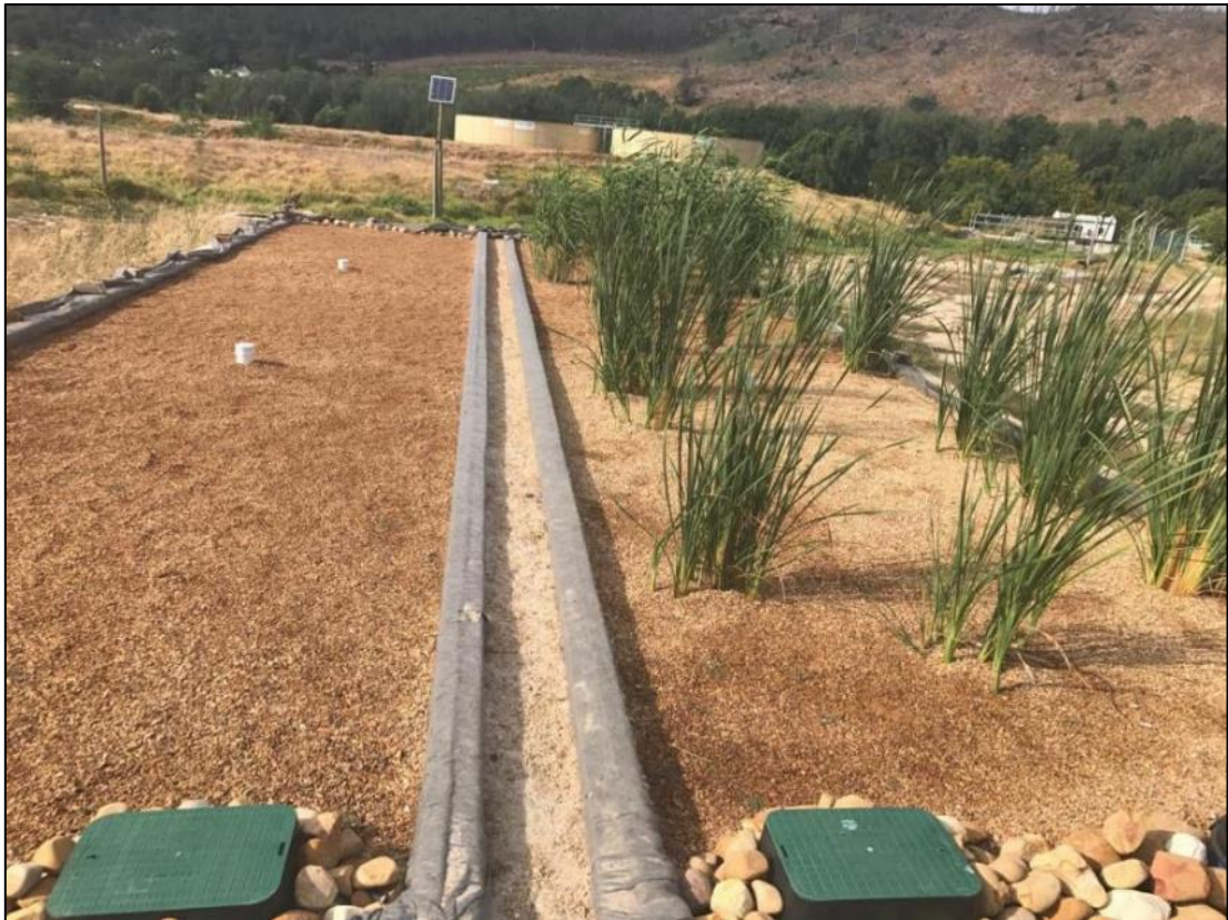
Biofiltration cells: SS (left) and SSV (right)
