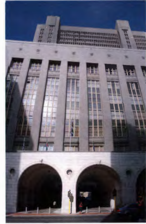
Fig 06 : Provincial Legislature, Western Cape Building:
