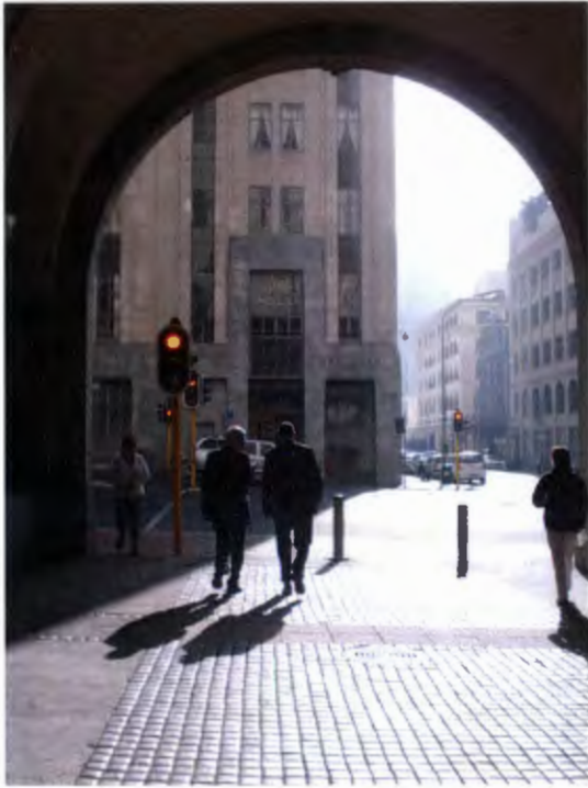
Fig 04 : Provincial Legislature building on Wale Street, A gateway to the Law Chambers , and High Court in Keerom St
