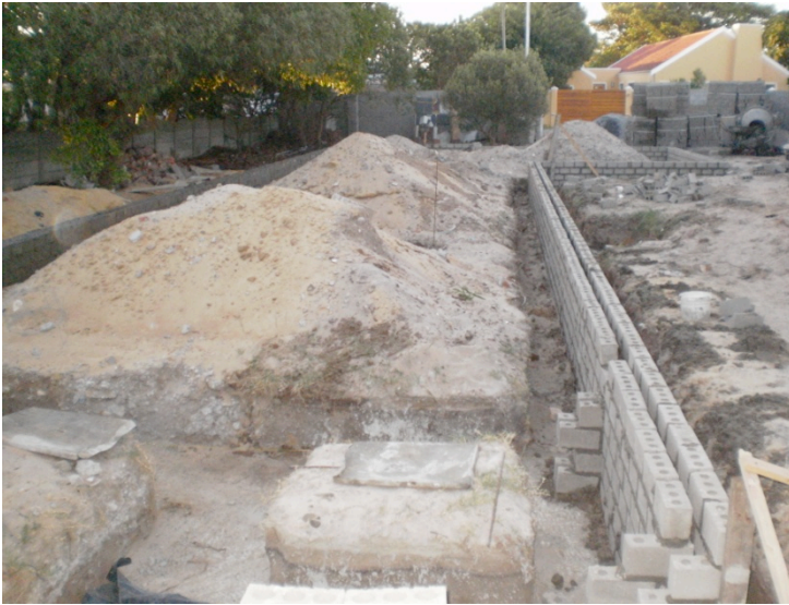
Figure 20a. Foundation wall construction Source: CON1018W 2010 Group 11
