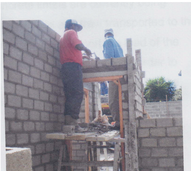
Masonry Wall Under Construction
