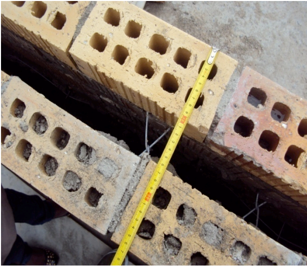
Cavity wall construction
