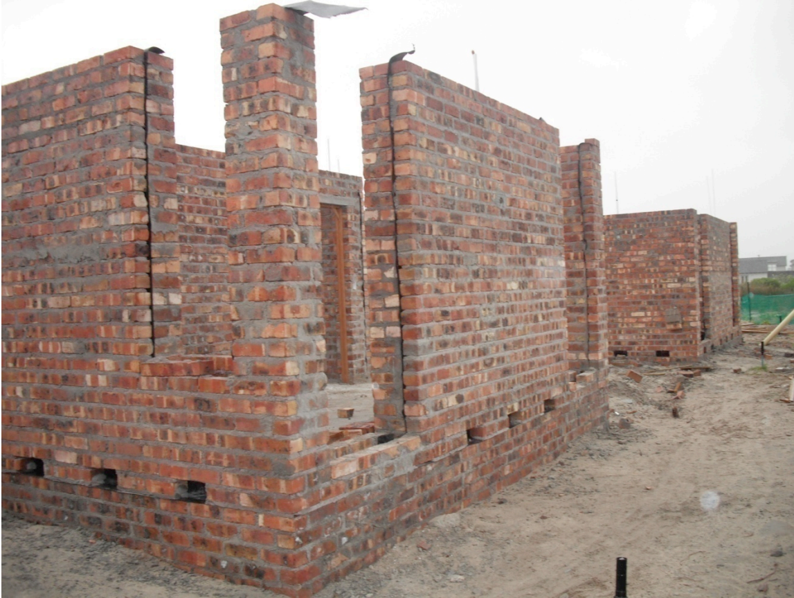
Cavity Wall Under Construction
