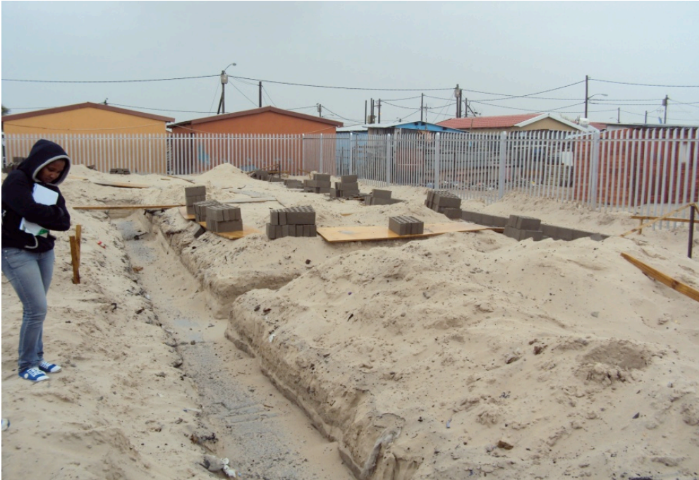
Figure 19a. Trench Excavation Source: CON1004W 2010 Group 2
