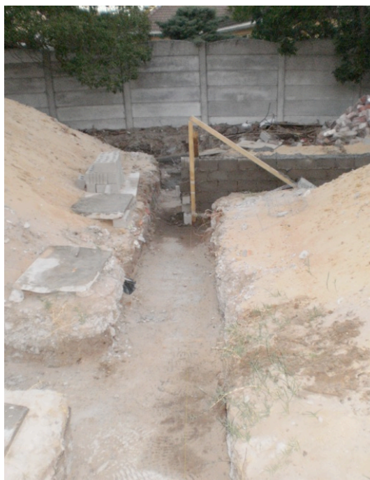
Figure 19b. Trench Excavation Source: CON1018W 2010 Group 11
