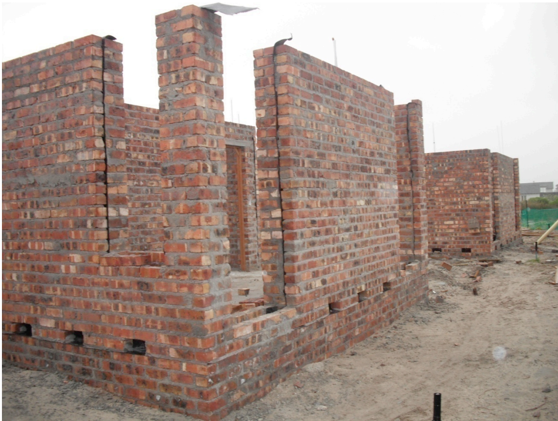
Picture showing weep holes Source: CON1004W Group 8 Project Report
