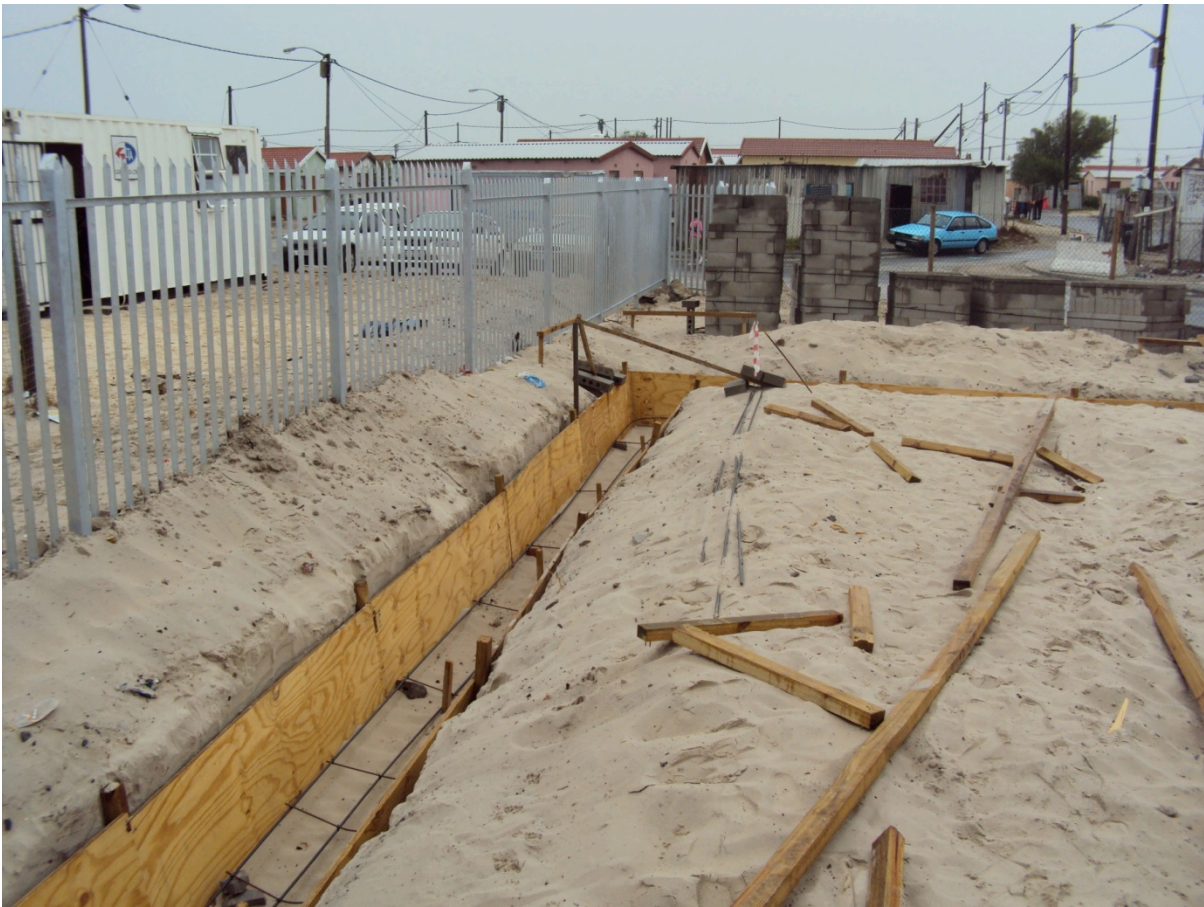
Figure 19 e. Earthwork support Source: CON1004W 2010 Group 2
