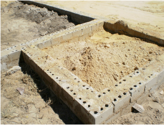
Figure 20c. Foundation construction Source: CON1018W 2010 Group 11
