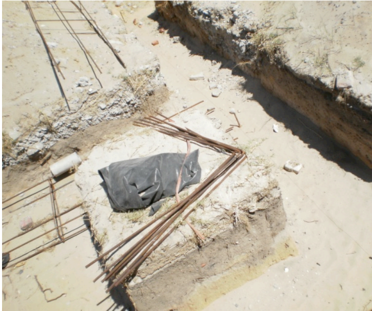
Steel Reinforcement Source: Group 11 CON1018W 2010)
