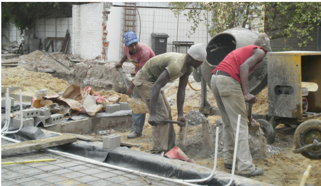
Figure 21: Concrete Fabrication Source: CON1018W 2010 Group 11
