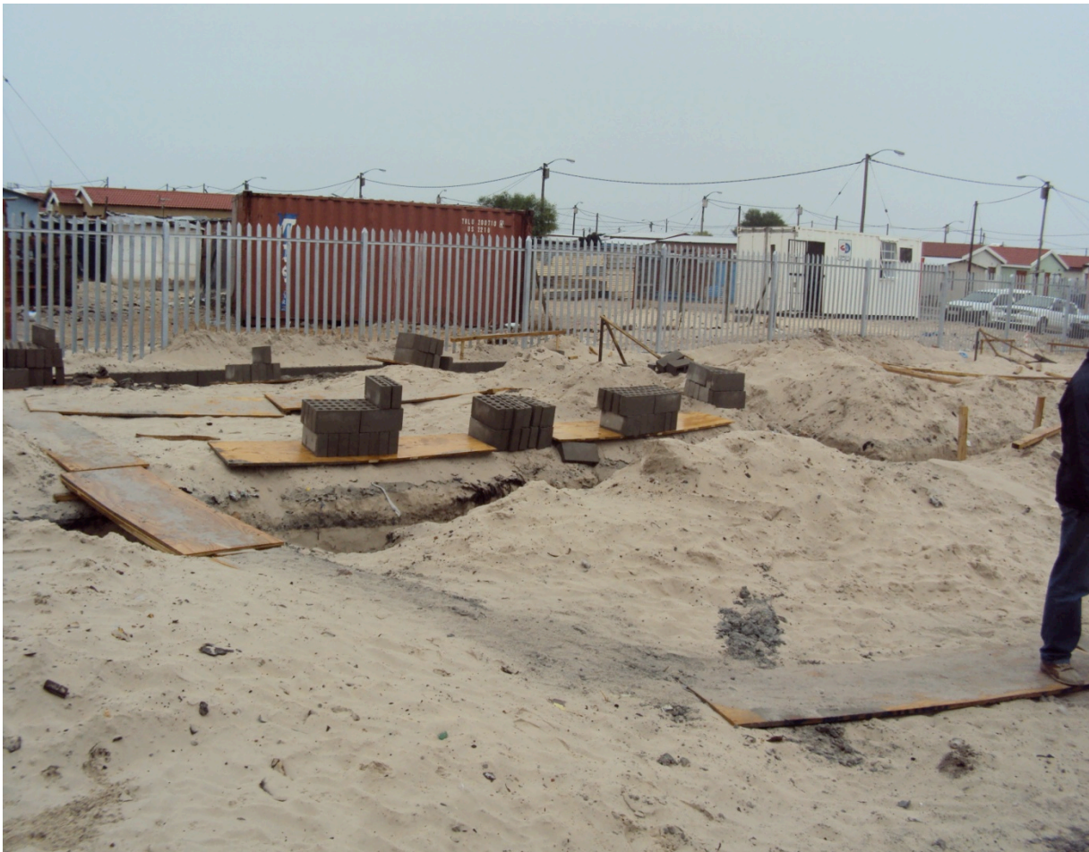
Figure 19 c. Trench Excavation Source: CON1004W 2010 Group 2
