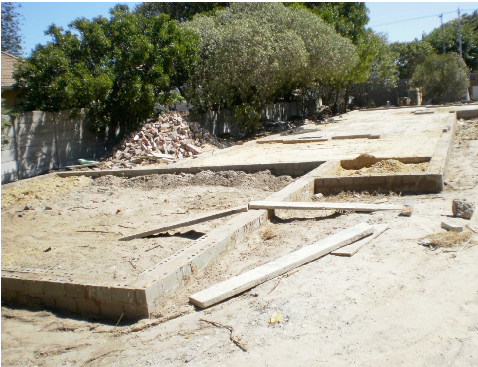
Figure 20b. Foundation construction Source: CON1018W 2010 Group 11
