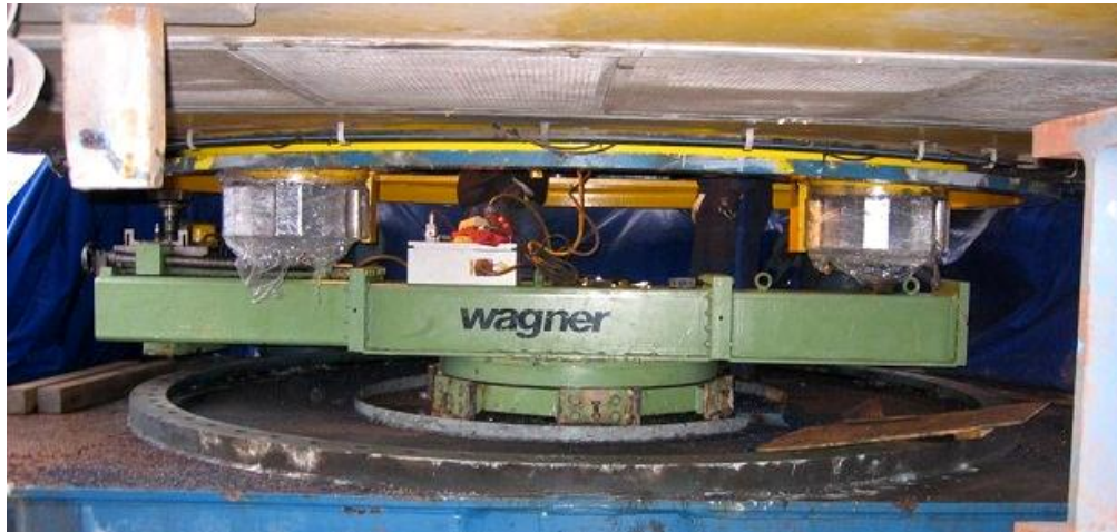
Figure 32: Inverted milling of a harbour crane upper bearing seating.
