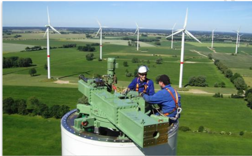
Figure 4: A circular milling machine operating on an installed wind tower.
