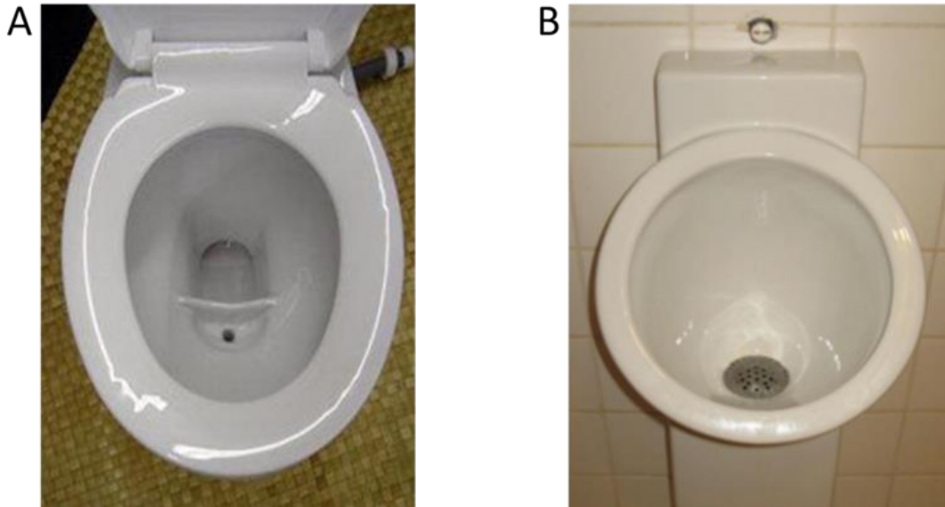
Figure 1: (A) No-mix toilet (Anand and Apul, 2014); (B) Waterless urinal (Münch and Dahm, 2009).
