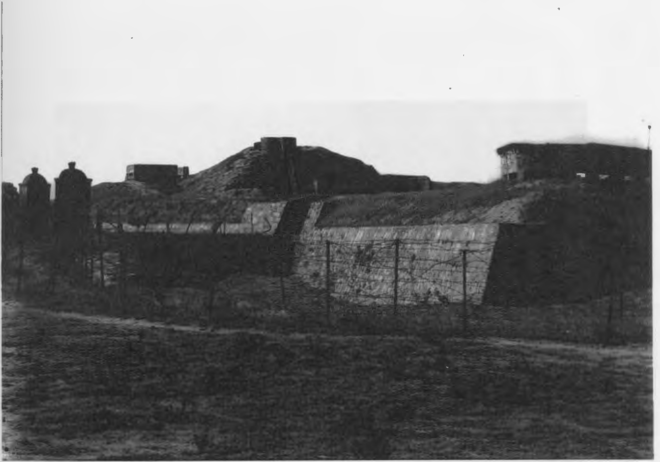
Figure 9: Fort Knokke, ca. 1910-1920 (De Smidt, no date)
