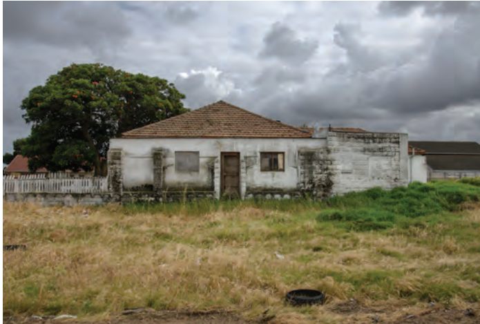
Fig 18 - Abandoned House, Cravenby. 2013.
