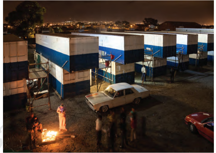
Fig 23 - Temporary Housing during the Upgrading of Social Housing, Eureka. 2013.
