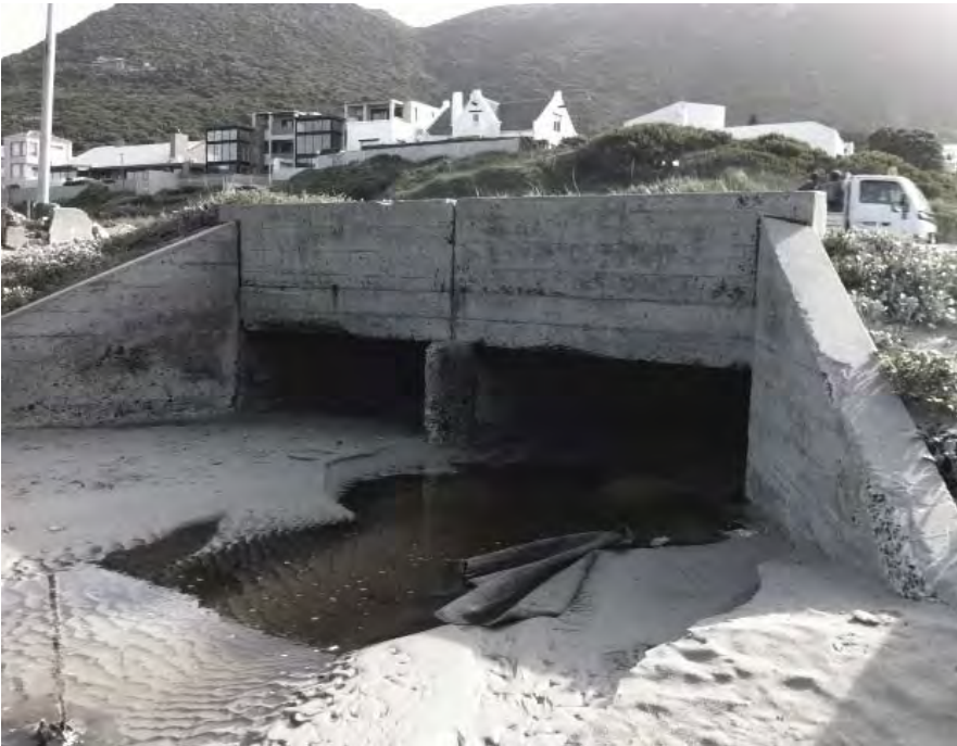
Fig 49: Existing tunnel for the river and sand flow
