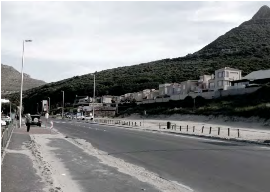
Fig 29: 2014: Sand overflowing on to the road
