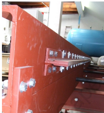
FIGURE 5-24: PHOTO SHOWING THE BOLTS ATTACHING A RAIL TO ITS SUPPORT
