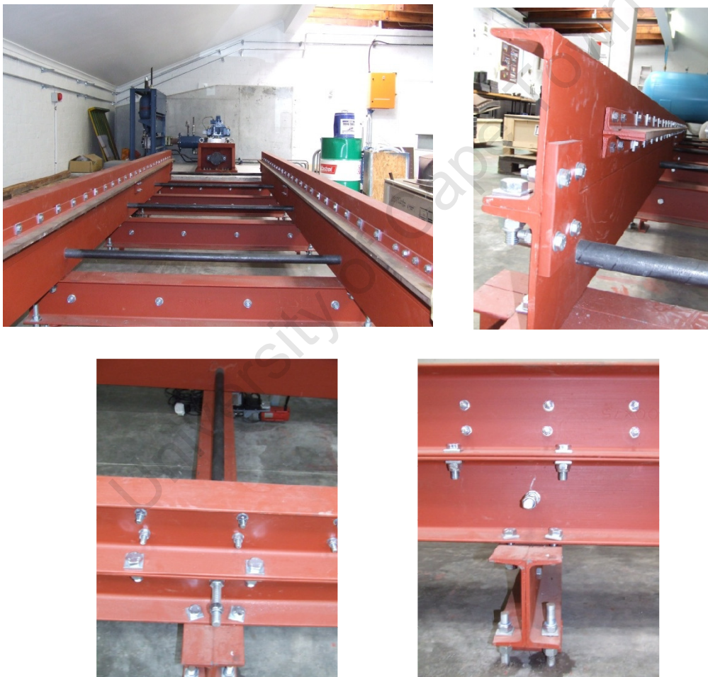
FIGURE 5-1: PHOTOS SHOWING THE CONSTRUCTION OF THE RAIL SUPPORT STRUCTURE
