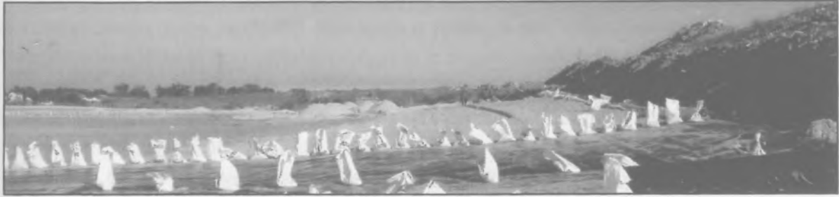
Figure 3.8 Belleville South Landfill liner slope
