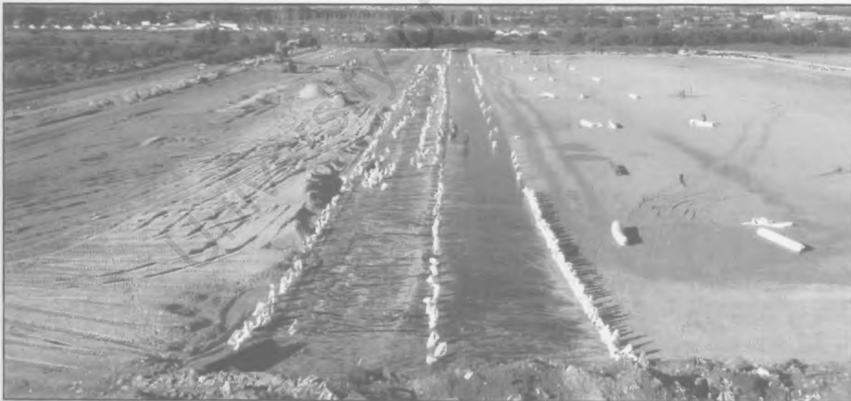
Figure 3.6 Bellville South Landfill liner system installation
