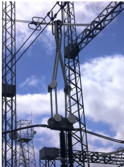
Figure 2.5 Pantograph type of disconnector [Courtesy of Eskom]
