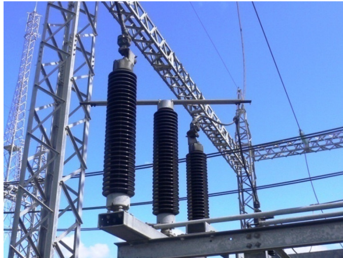
Figure 2.4 Double break type disconnector [Courtesy of Eskom]
