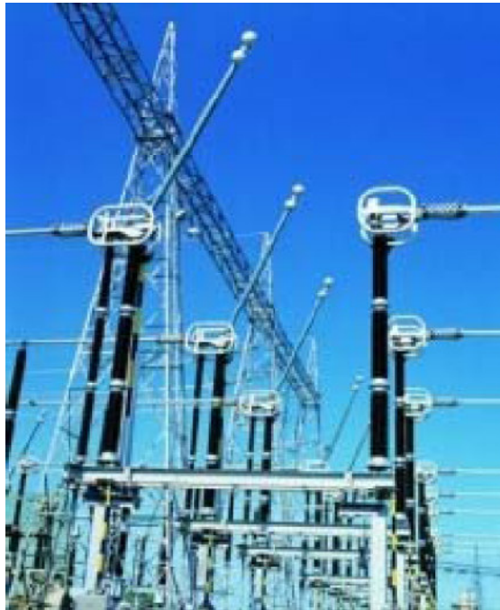
Figure 2.2 Vertical Break type disconnector [4]
