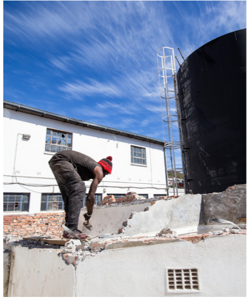
Fig. 47 - Man knocking out bricks at Oceana plant (Hendricks, 2022)
