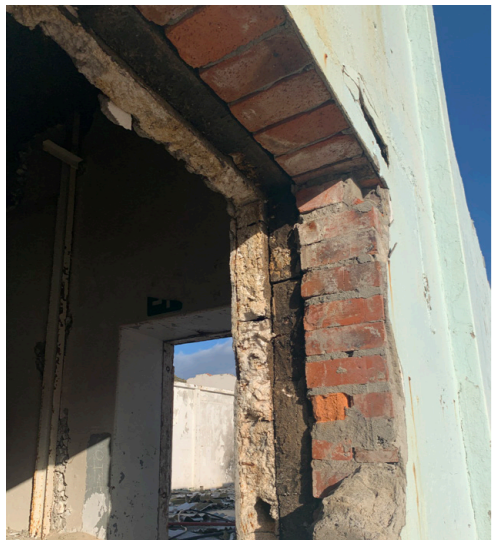
Fig. 117 - 230 brick wall, with a 100mm (Author, 2022)
