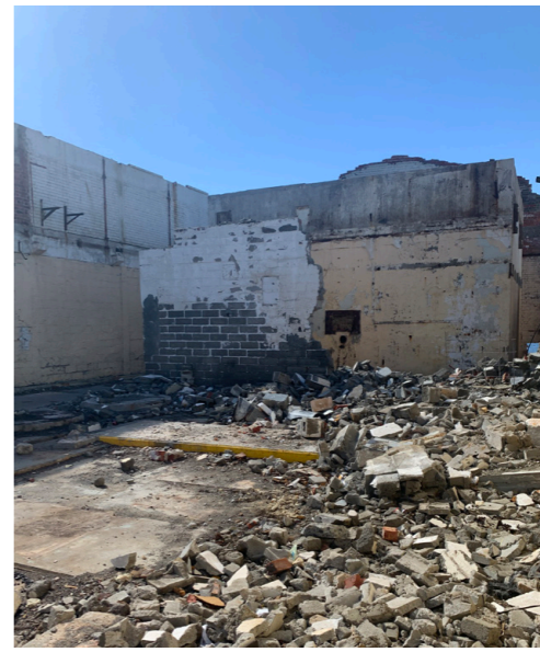
Fig.48 - Rubble in the ruin (Author, 2022)
