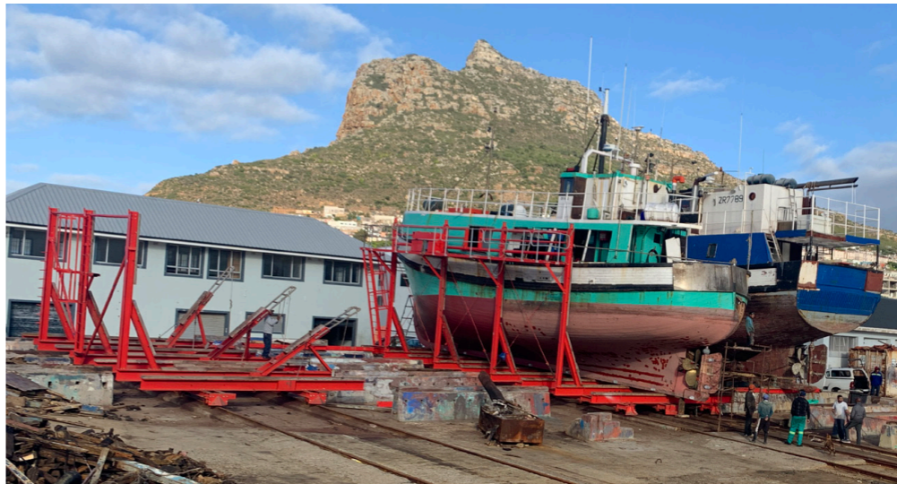
Fig. 123 - The steel support structure in the drydock used to keep boat stable and acts as scaffolding to fix boats. Learning from the existing form follows function. (Author, 2022)
