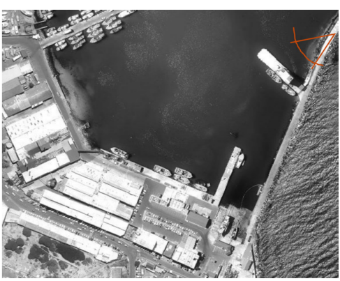
The ice factory in the foreground with the fishmeal plant and Hangberg in the background.
