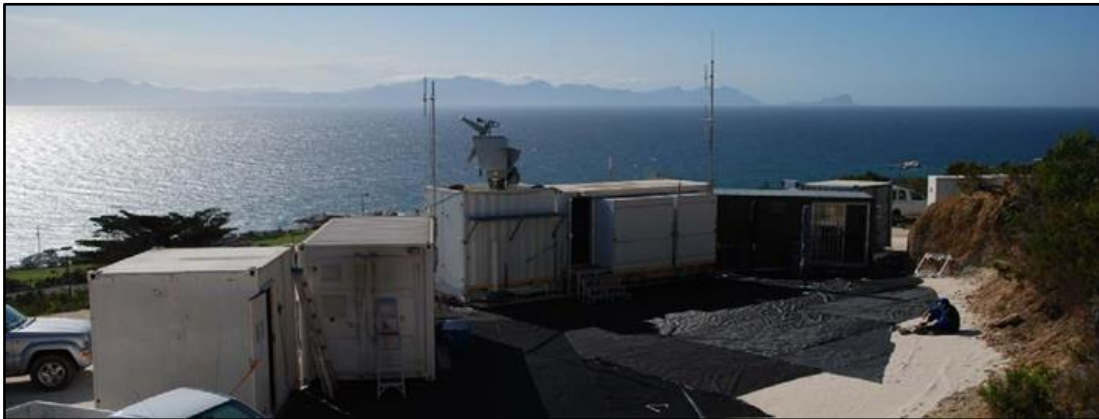
Figure 3.1 Experimental multimode radar deployed in Simons Town [35]
