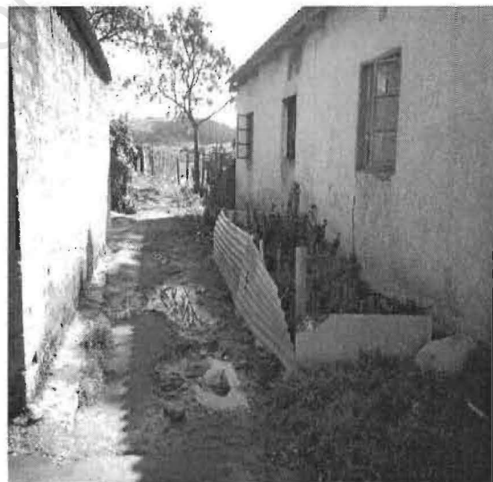
Figure 4: Stagnant water from leaking and polluted tap. People use tap water.
