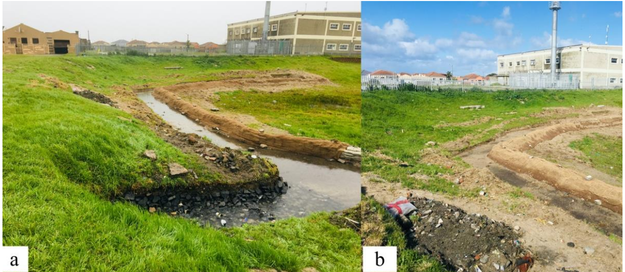
Figure 6-13: a) Ponded infiltration swale after a storm, 26 August 2021 (16:51) b) Dry infiltration swale, 27 August 2021 (10:35)
