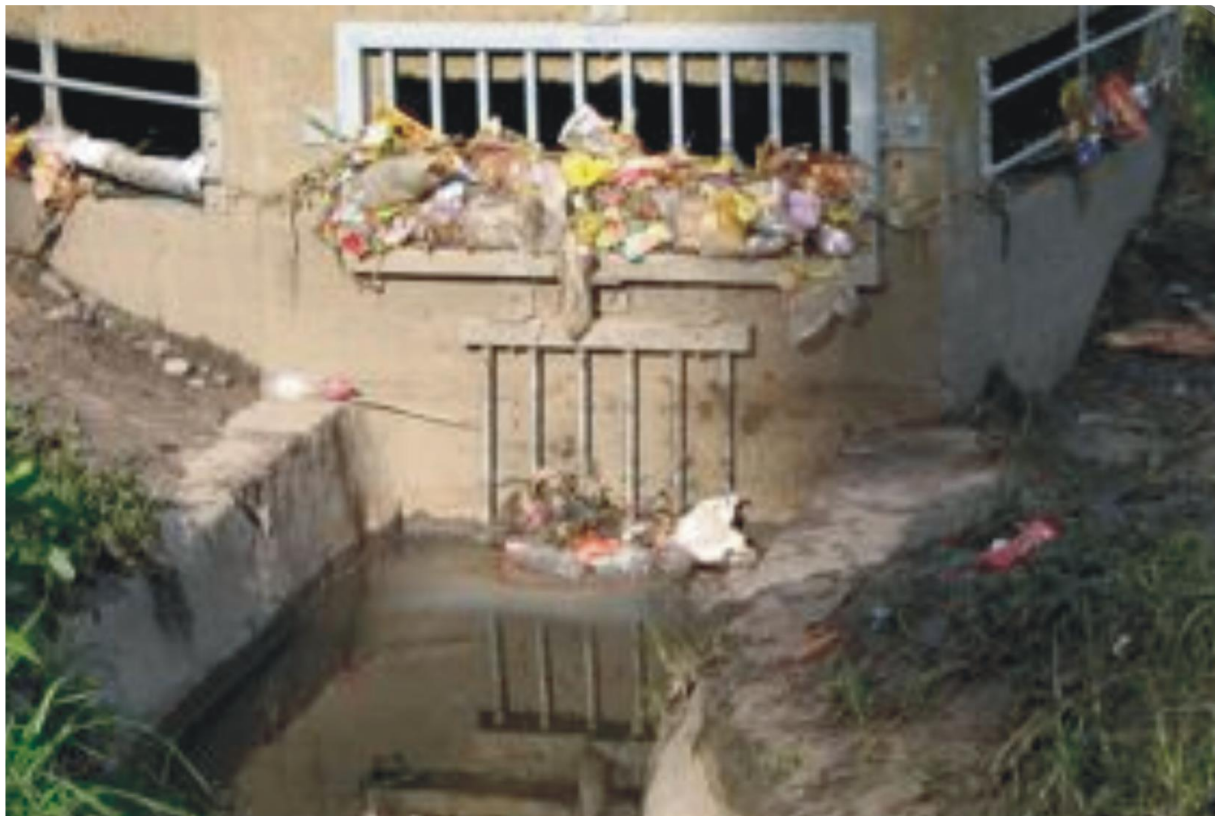
Figure 2-7: Litter build-up at one of the stormwater inlets in the AWRMS (Department of Water Affairs, 2010)
