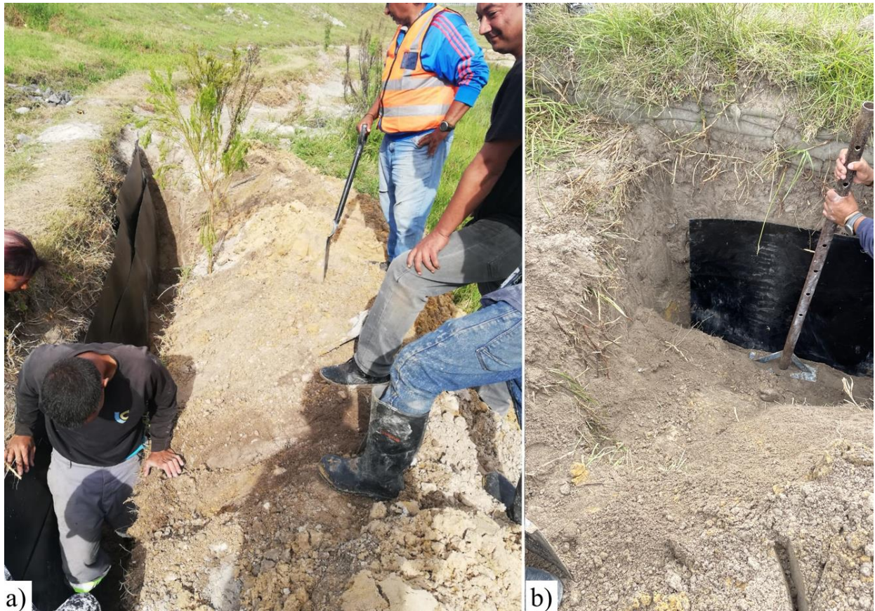
Figure 6-20: a) placing the mole barrier b) compacting the trench
