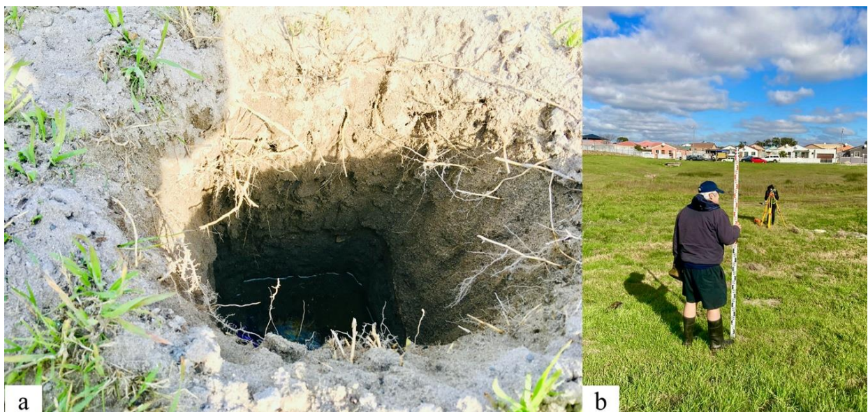
Figure 6-5: a) Trial pit b) setting out the berm line
