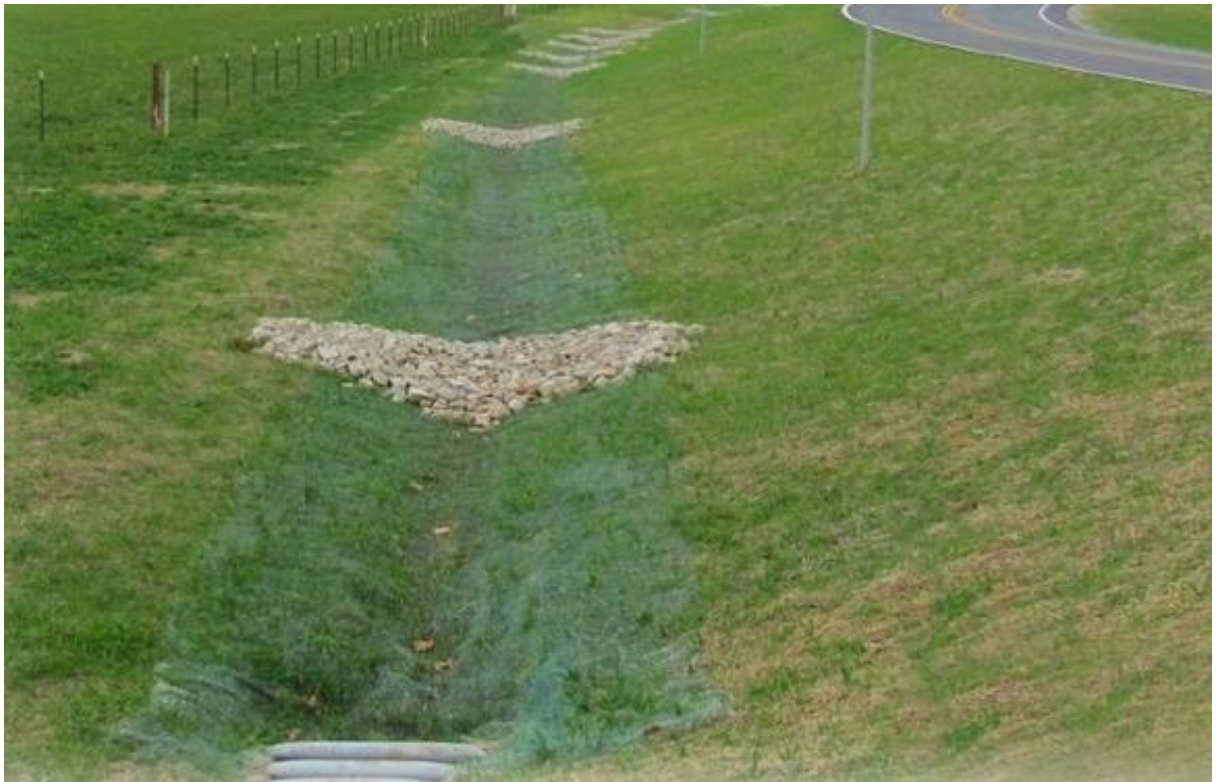
Figure 2-4: Top: Diagrammatic plan of an infiltration pond with forebay; Bottom: Rock check dams across a drainage ditch (Winston et al. , 2019)
