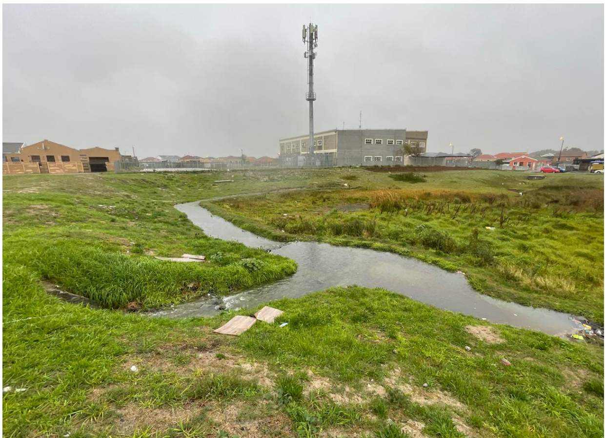
Figure 6-17: a) Full swale during a storm
