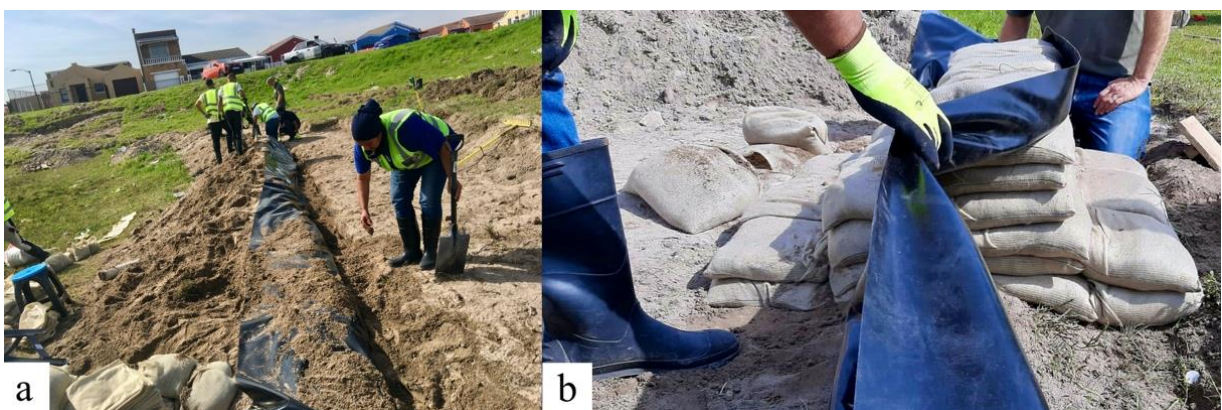
Figure 6-8: a) Residents positioning the PVC sheet b) Assembling the sandbag berm
