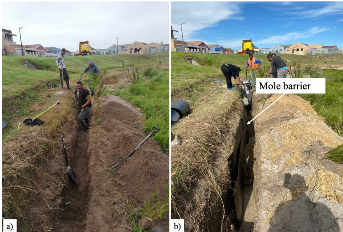
Figure 6-19: Excavating the trench for the mole barrier
