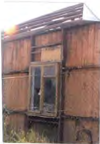
Figure 24. New window, west elevation
