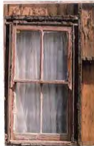
Figure 25. Original sash window, east elevation
