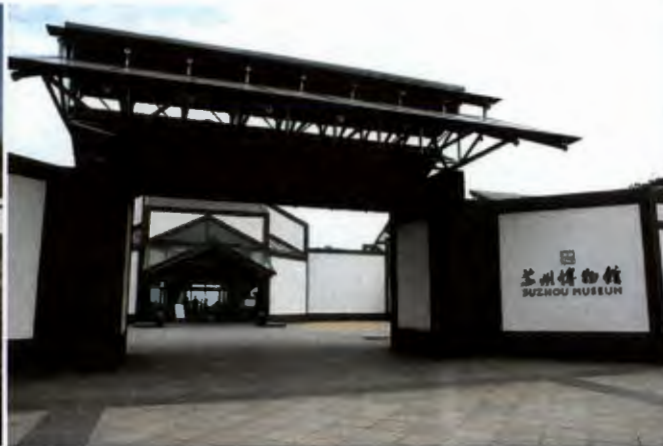
Middle: Steel structured canopy at the main entrance, representing the traditional Chinese roof.
