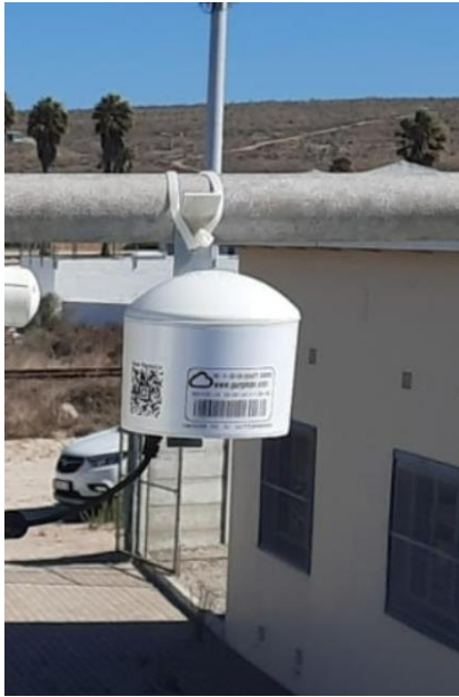
Figure 14: The PurpleAir Particulate Sensor installed at the Saldanha AQM Station
