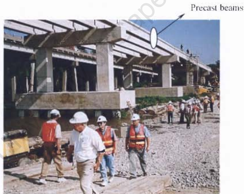
Fig 1.1: Concrete-concrete composite bridge under construction
