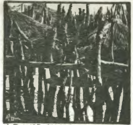
A PALISADE SHOWING THE BEAM FOR LATERAL SUPPORT.
