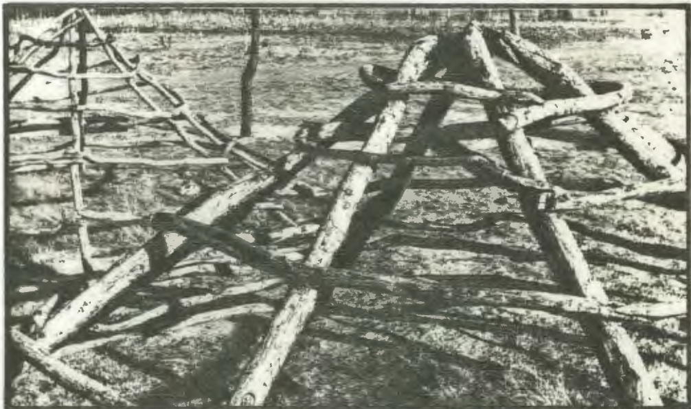
ROOF FRAME : MADE FROM MOPANI SAPLINGS.
