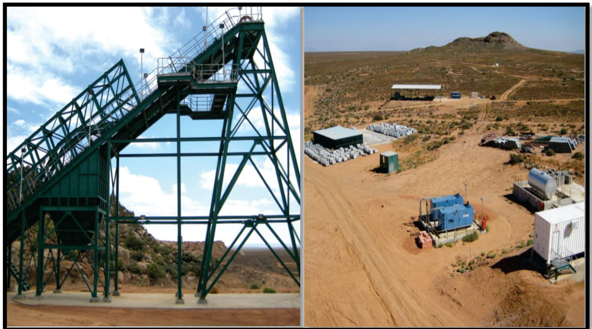
FIGURE 10: INCLINE SHAFT HEADGEAR AND STEENKAMPSKRAAL MINE SITE
