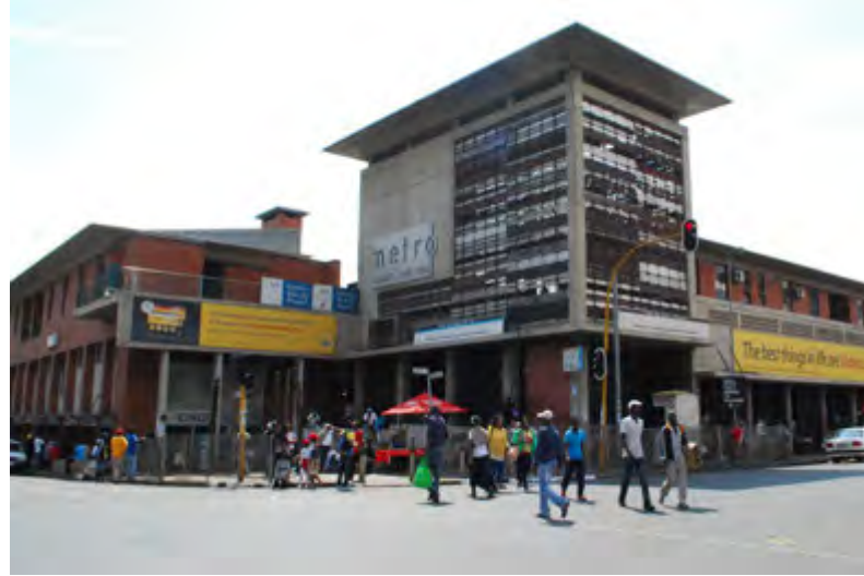
Figure 65: Metro Mall – Off Shutter Concrete + Bricks + Steel
