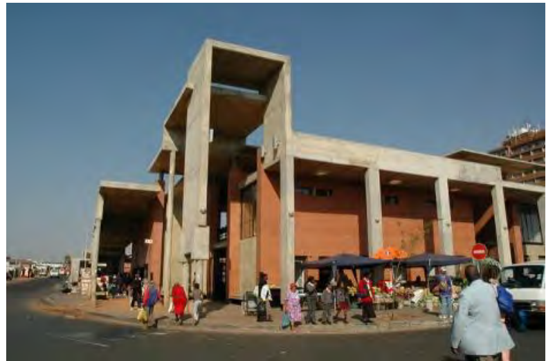
Figure 166: Exterior - Brick & off-shutter Concrete
