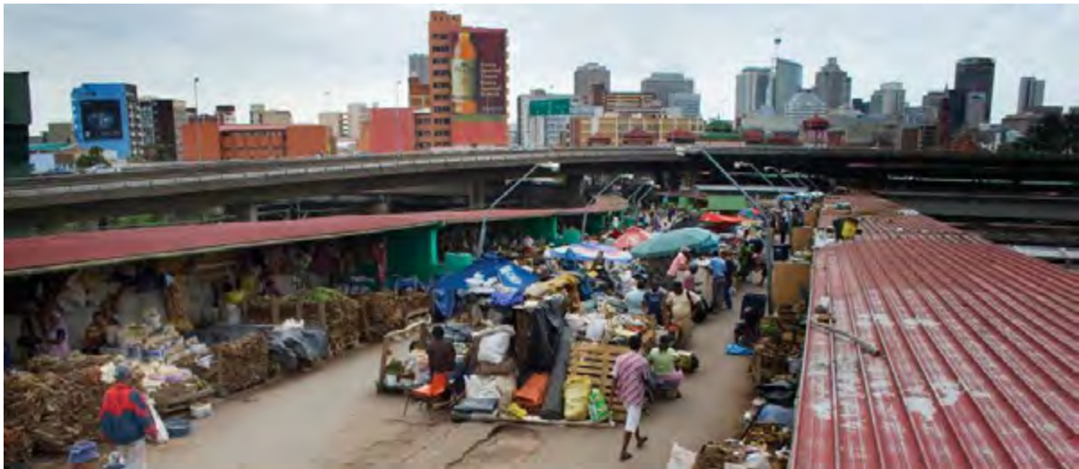
Figure 175: Muthi Market – New Steel Roofing
