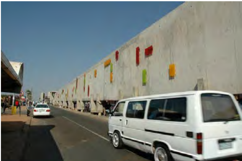
Figure 165: Exterior - off-shutter Concrete
