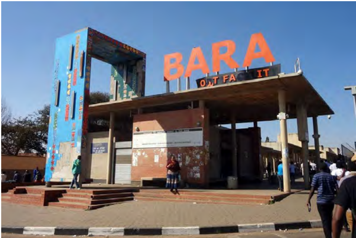
Figure 158: Baragwanath Transport Interchange and Traders Market – Baralink Main Entrance
