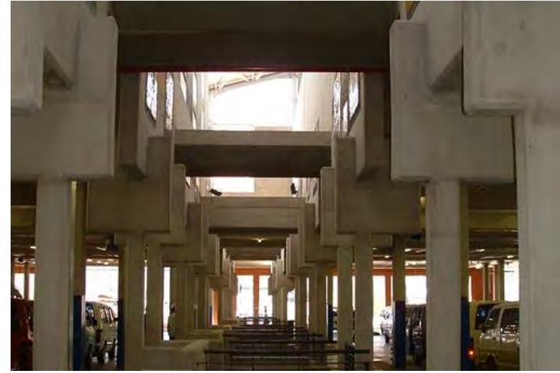
Figure 66: Metro Mall – Off Shutter Concrete
