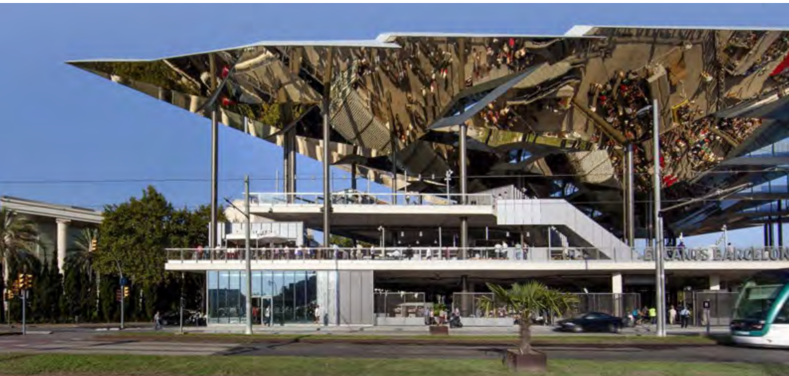
Figure 199: Escalator Connecting Intermediate Level to the Upper Level
