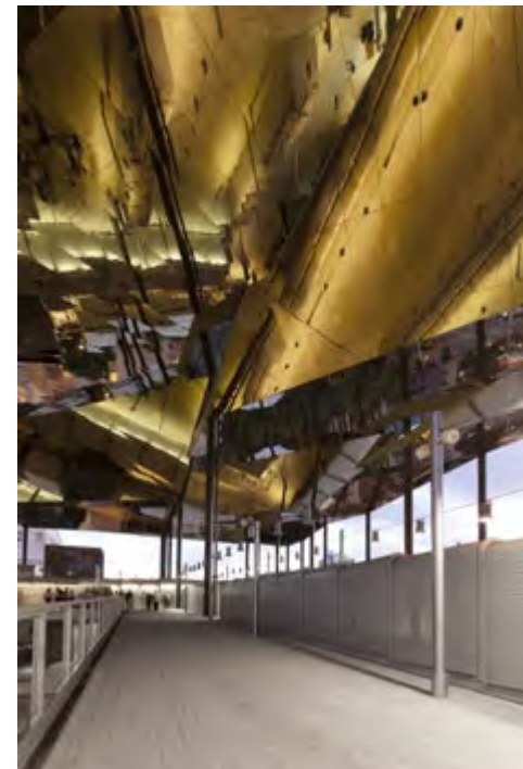
Figure 210: Roof Canopy – Interior
