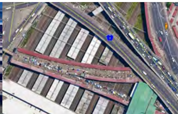
Figure 172: Unutilised Freeway After
