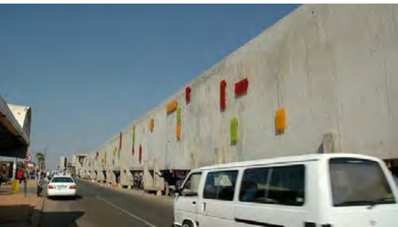
Figure 63: Baralink – Off Shutter Concrete
