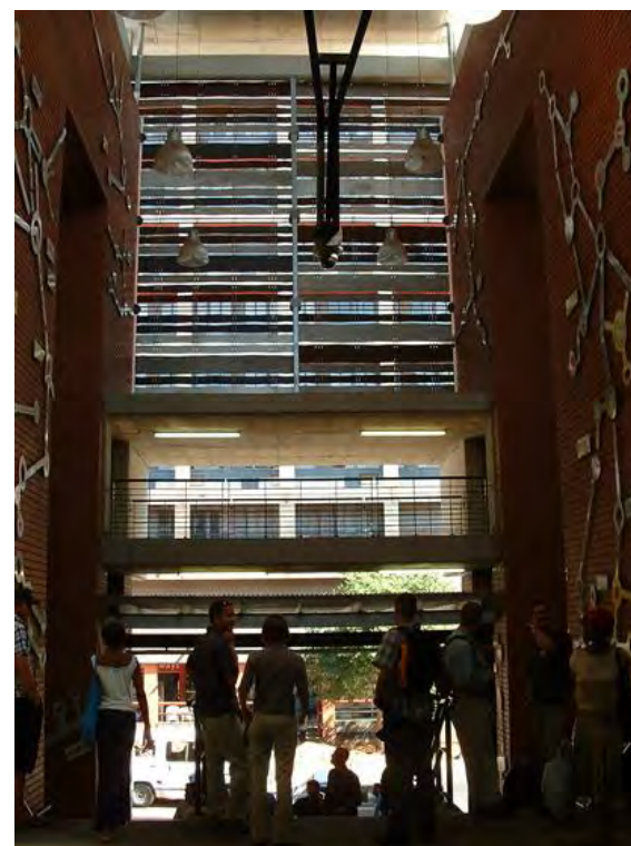
Figure 157: Oxidized Steel Screens
