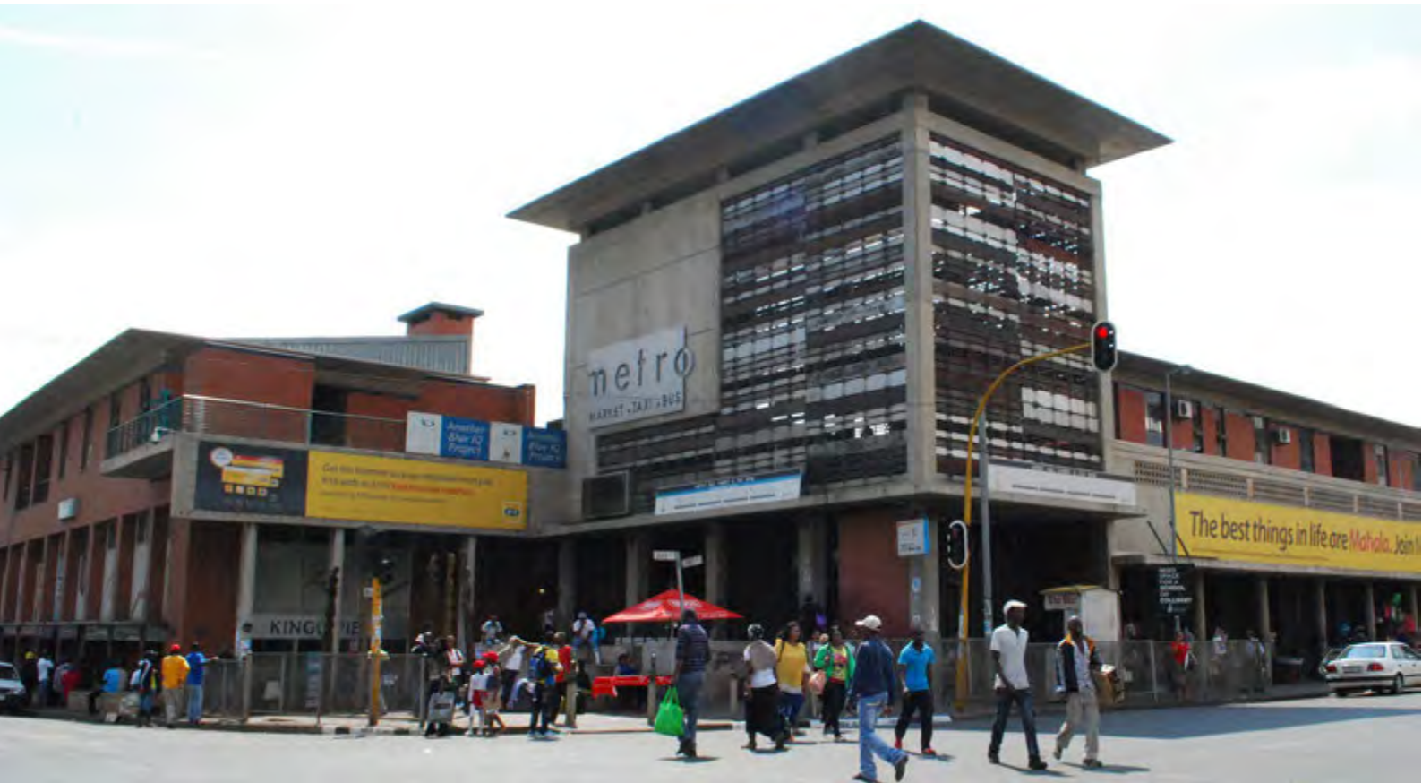
Figure 142: Metro Mall Transport Facility and Traders Market
