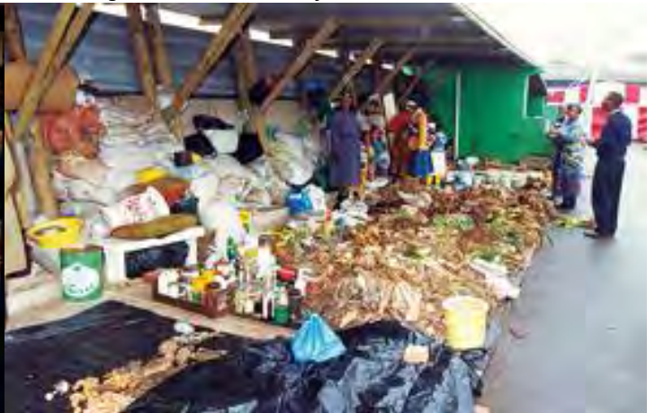
Figure 71: Muthi Market – New Steel Roofing
