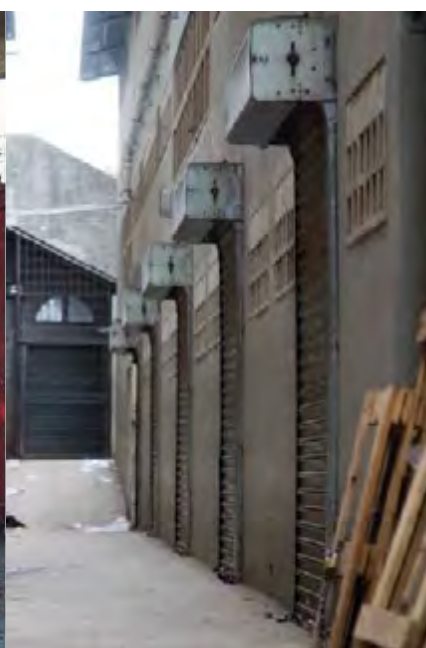
Figure 186: New trader storage facilities
