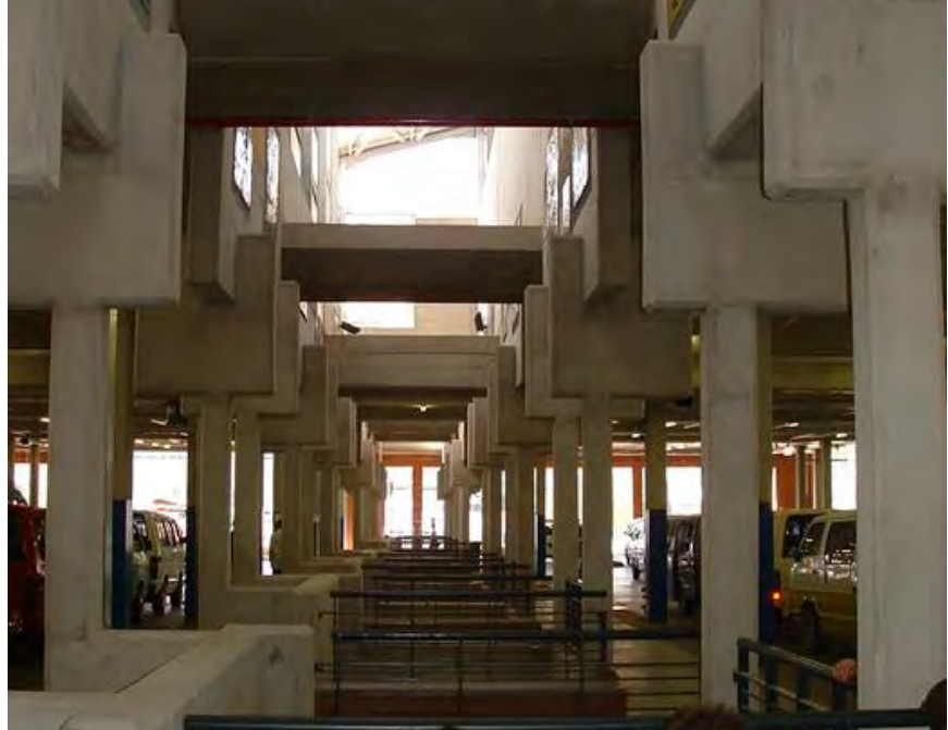
Figure 155: Off-Shutter Concrete Finish
