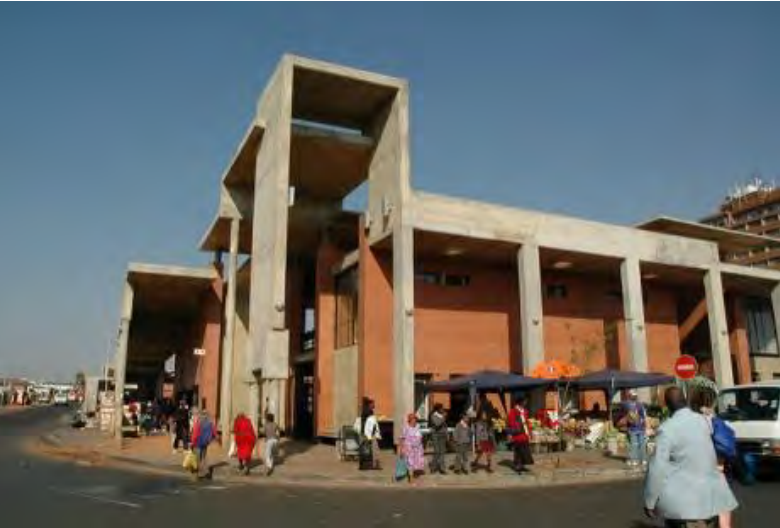
Figure 62: Baralink – Off Shutter Concrete + Bricks
