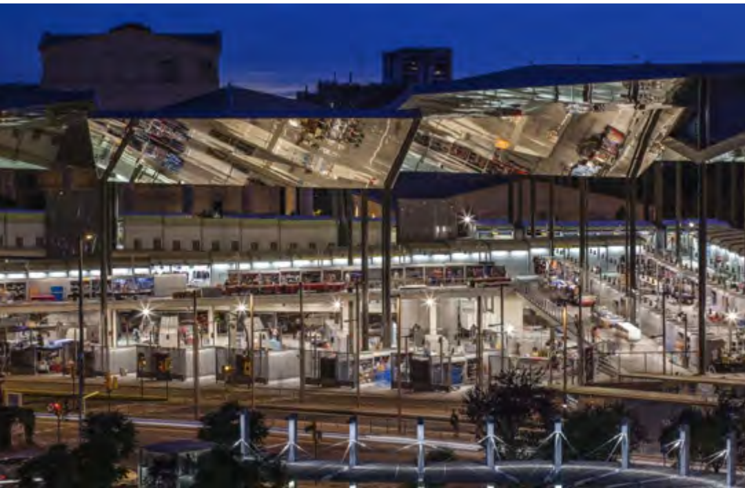
Figure 209: Roof Canopy – Exterior View
