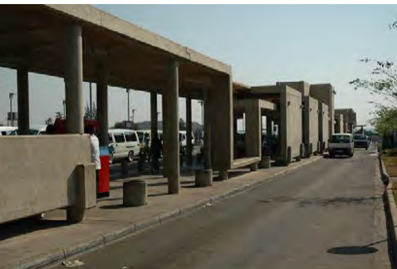
Figure 64: Baralink – Off Shutter Concrete
