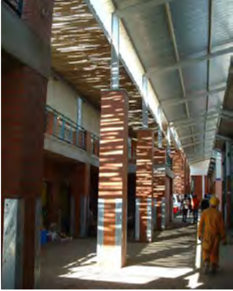
Figure 68: Metro Mall - Roof
