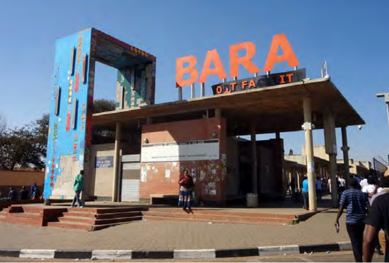
Figure 61: Baralink – Off Shutter Concrete + Bricks + Mosaics
