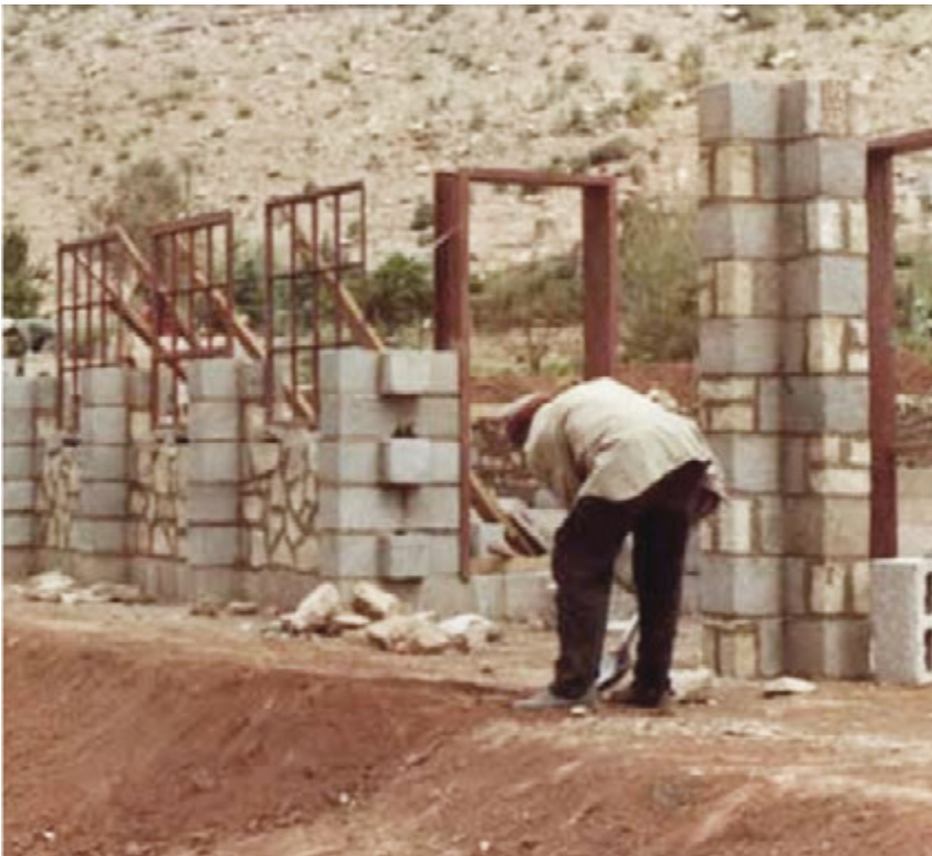
[57] A Lesotho School in construction.
