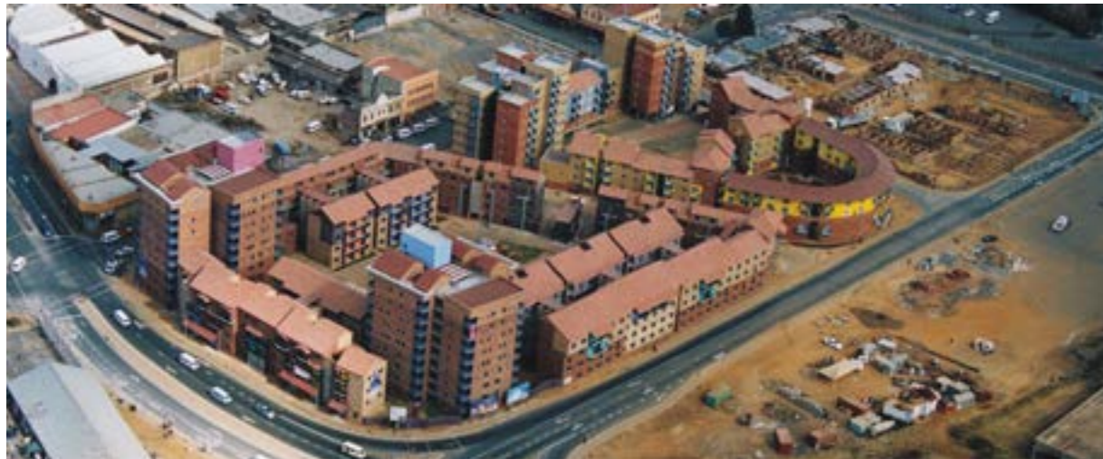
PHOTO OF BRICKFIELDS DEVELOPMENT Figure 4.1
