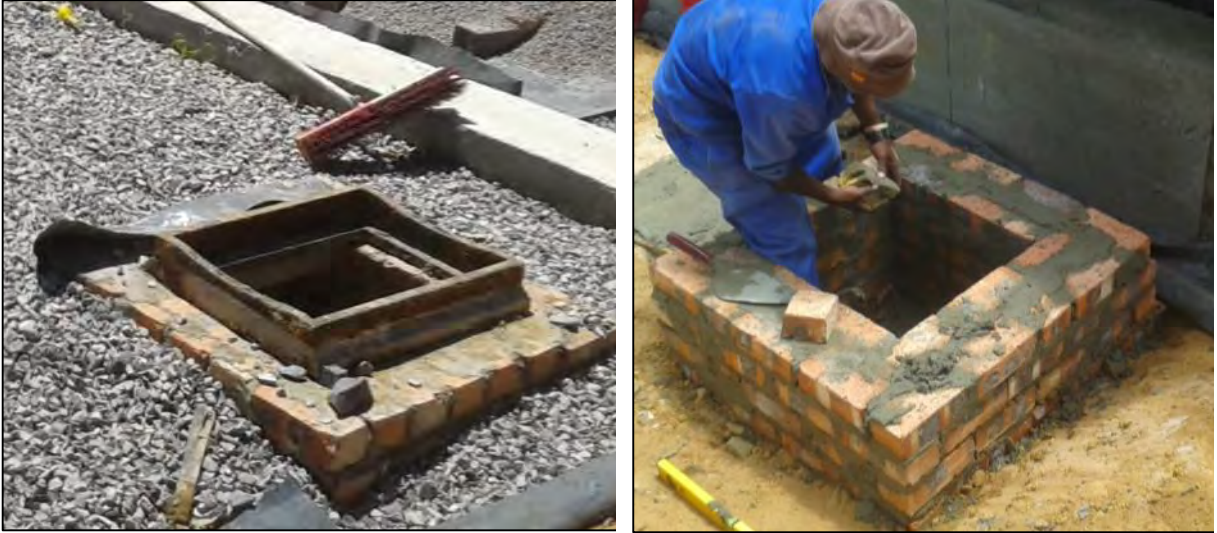
Figure D-5: Construction of NEB parking area monitoring chambers
