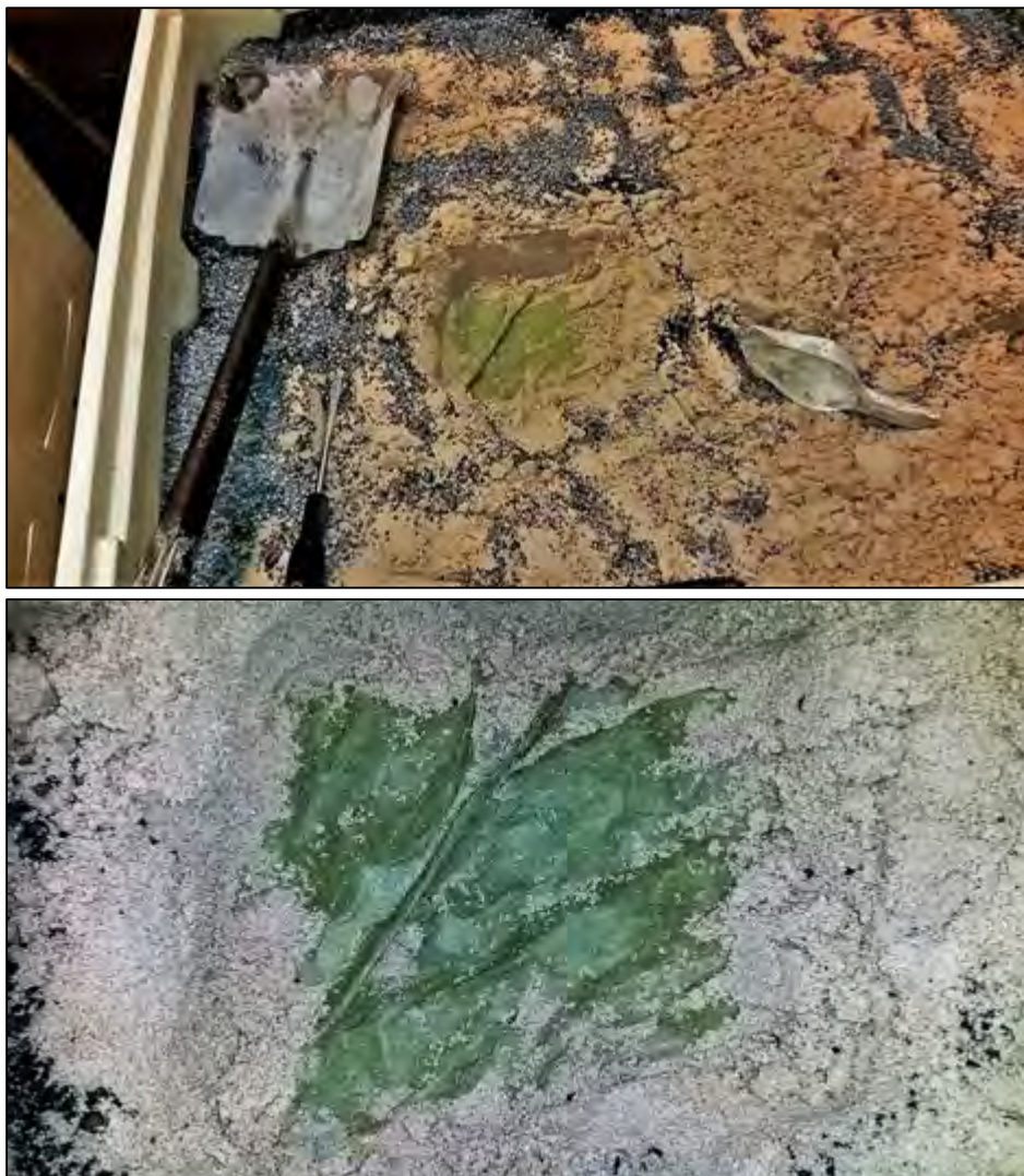
Figure 4-25: Excavation of the Inbitex® geotextile below the bedding sand
