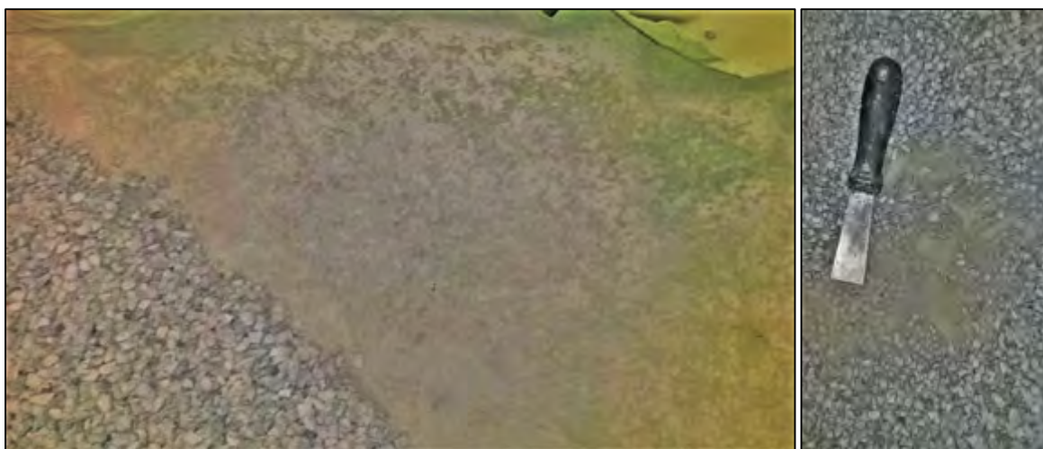
Figure 4-22: Excavation of Pavement B revealing the condition of the Inbitex® geotextile
