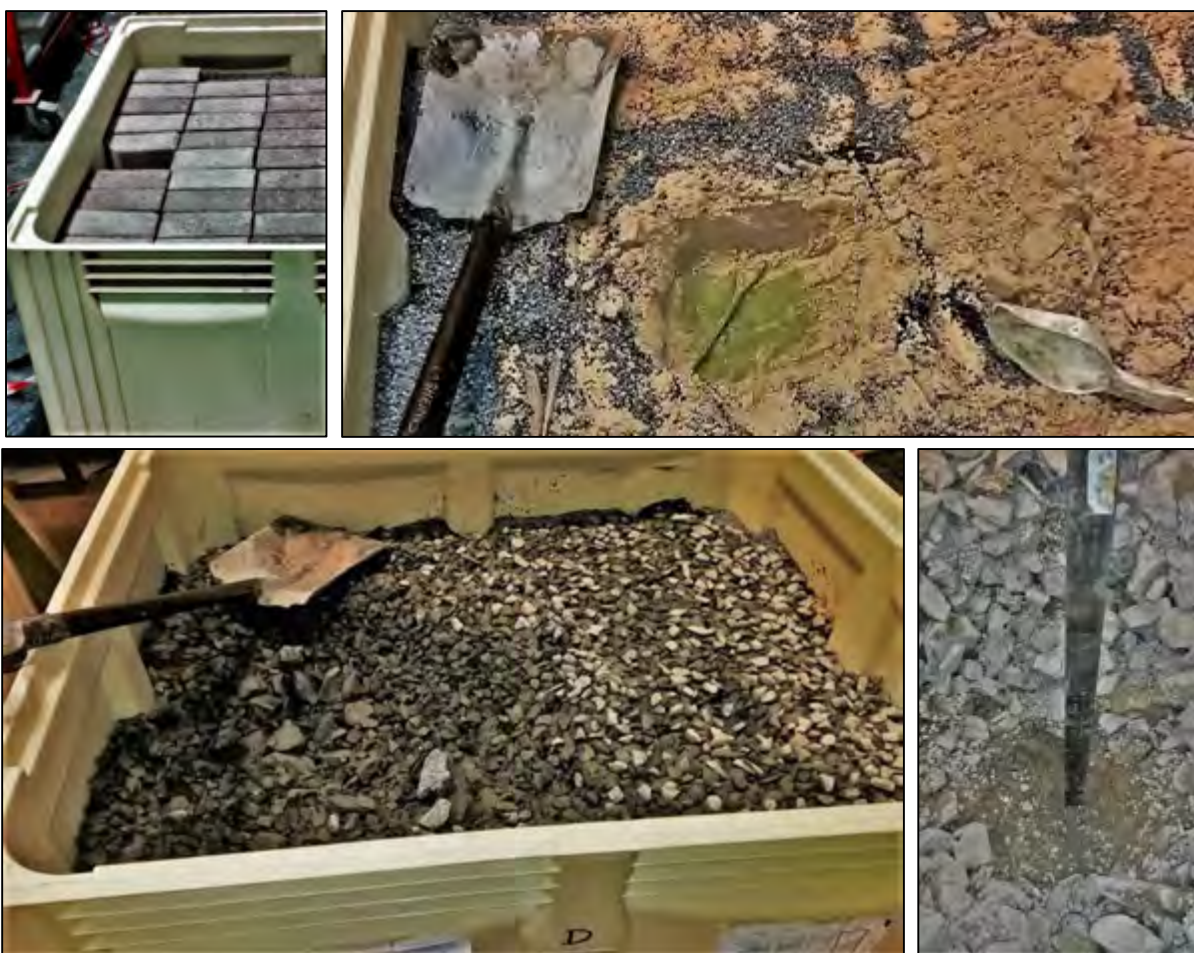
Figure 4-18: Pavement excavation documenting the internal condition of each structure
