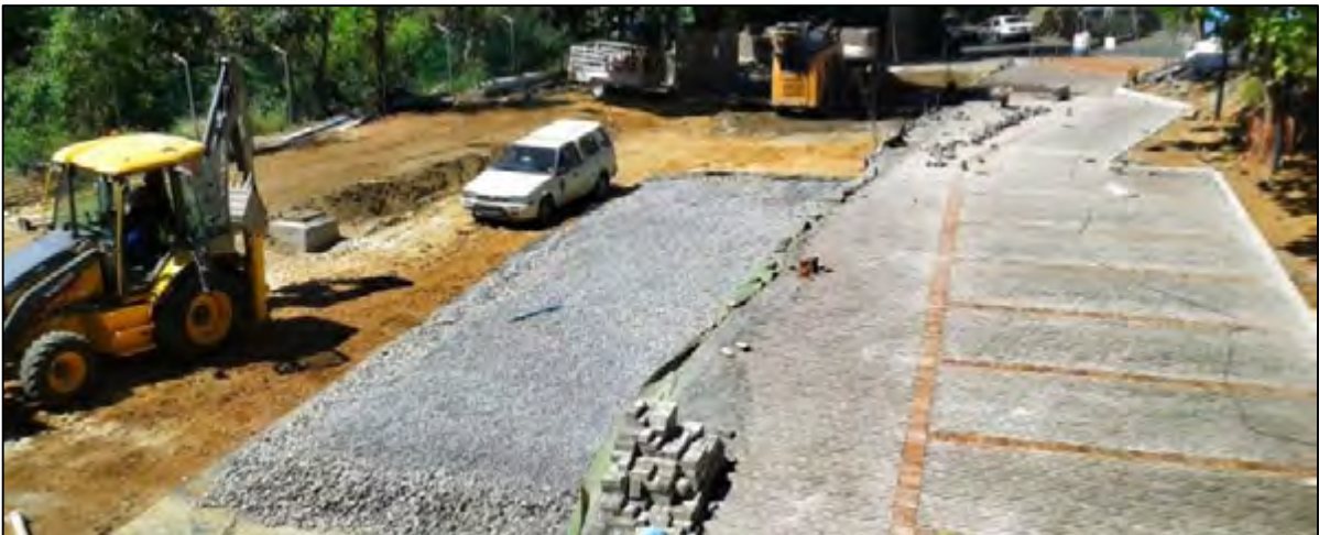
Figure D-10: Start of the second stage of construction
