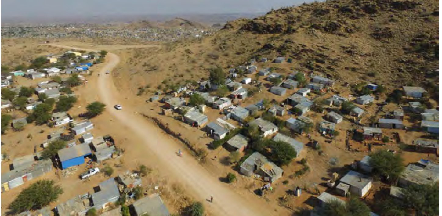
South West View down the main road
