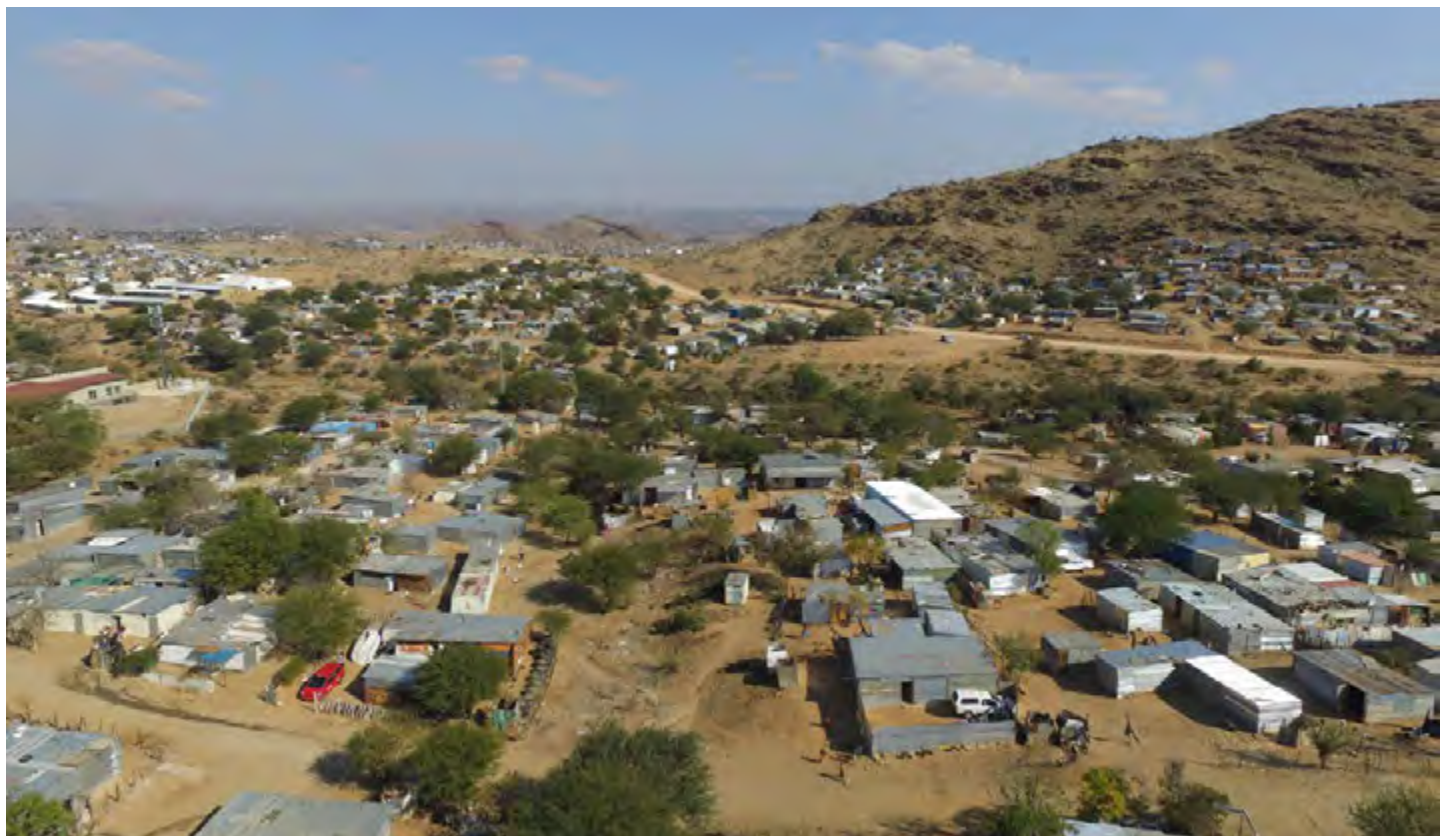
South West View down a tributary. In this photo one can notice the extent of informal toilets along this route. Although it is believed some are connected to the current over flowing sewer.
