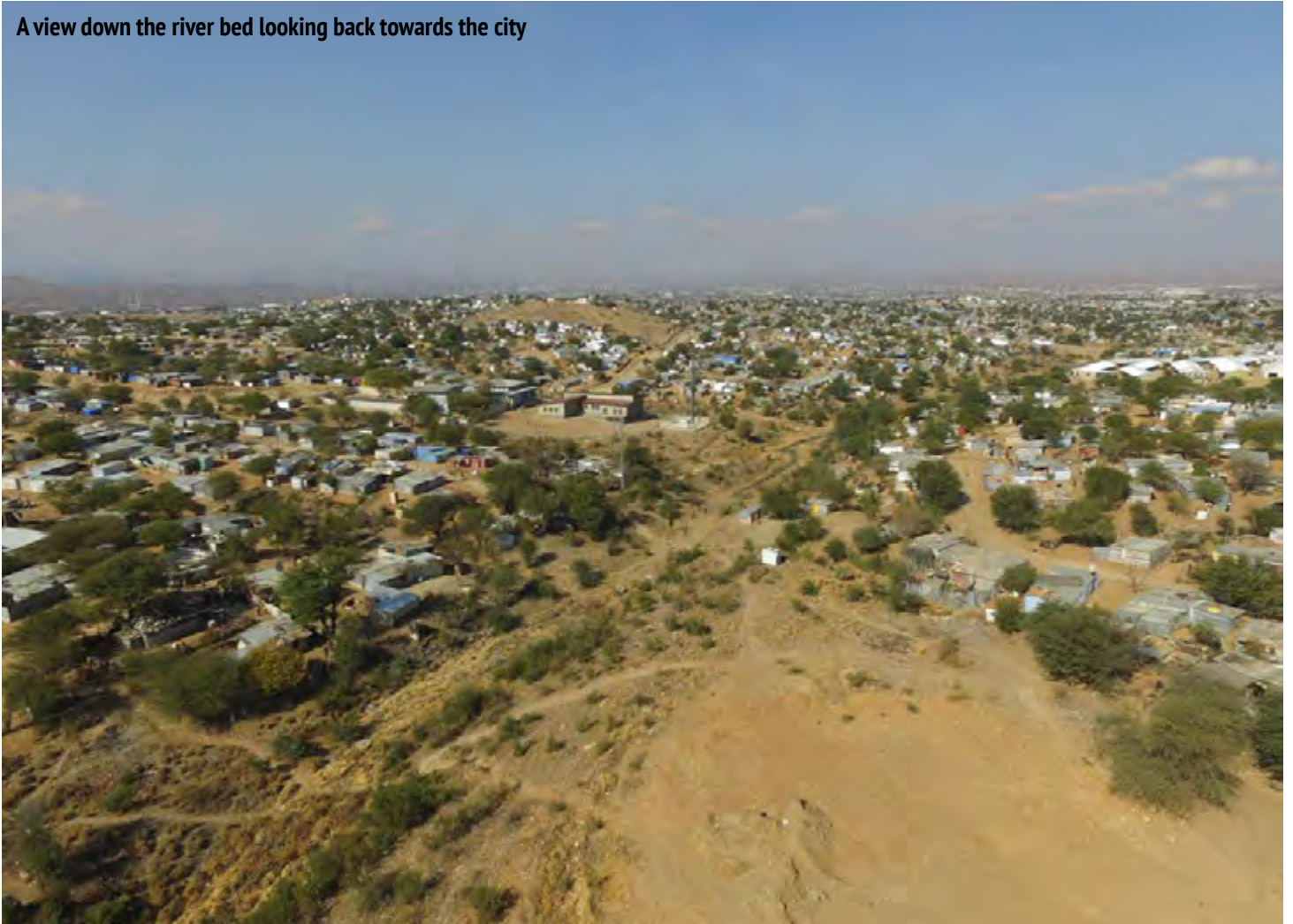
A view of the site in relation to the babilon fire station
