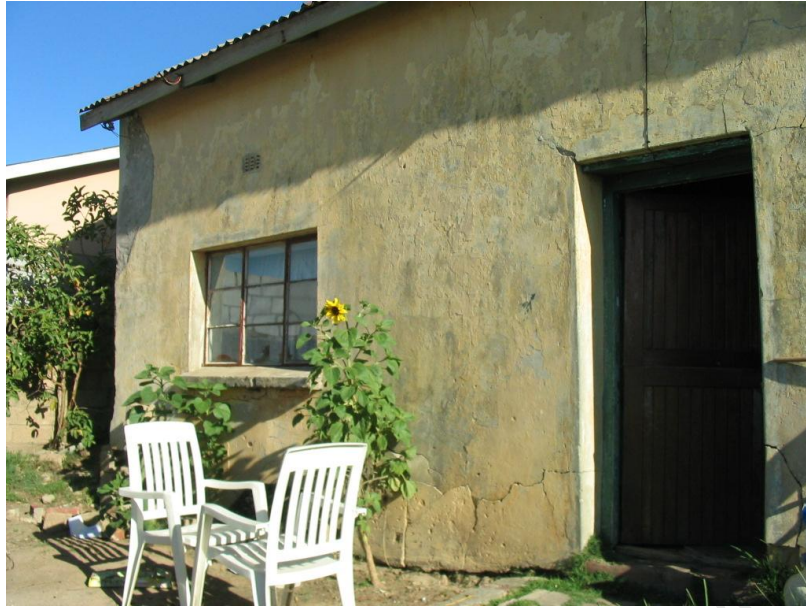
Fig 22: Original front façade of the dwelling, now the backdoor
