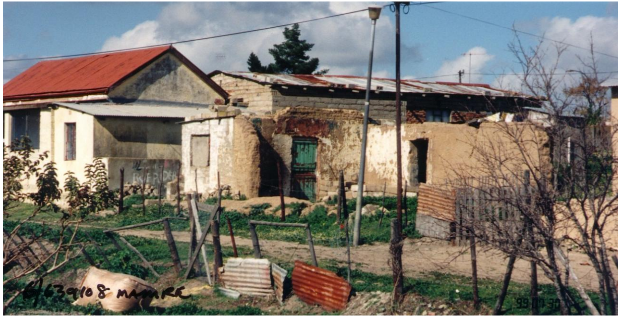
Fig 31: Three buildings showing various states of intervention – cement brick, corrugated iron, a modern lean-to and a ruin in the foreground (Rennie & Scurr, 1999)
