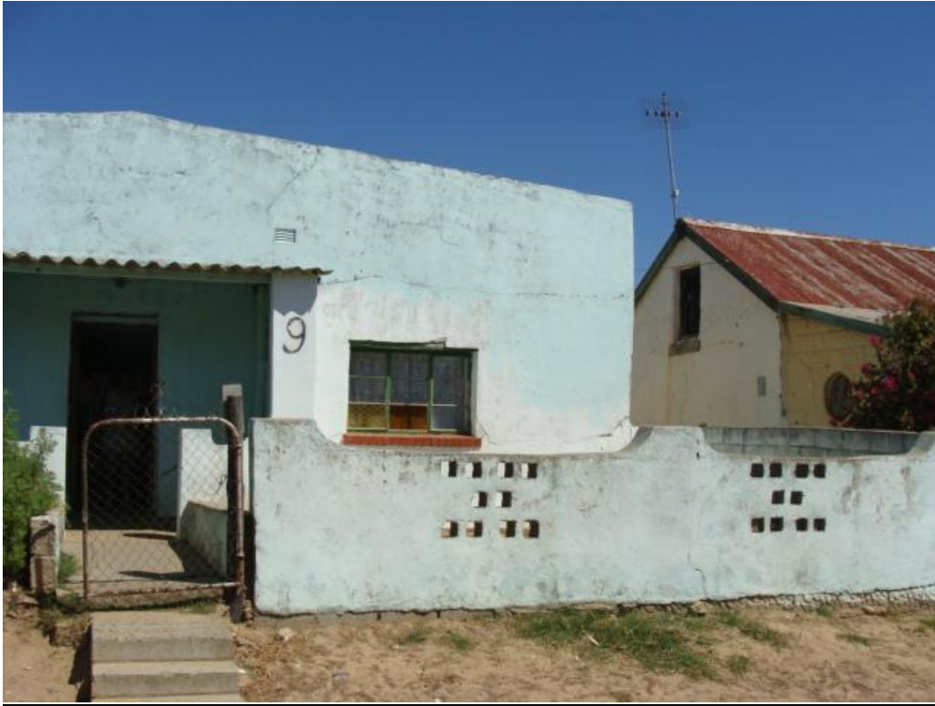
Fig 16: The Tituses' Dwelling in Adonis Street. Note the dwelling on the right is of correct proportions while the roof pitch on the Titus dwelling has been turned and made almost flat during insensitive alterations
