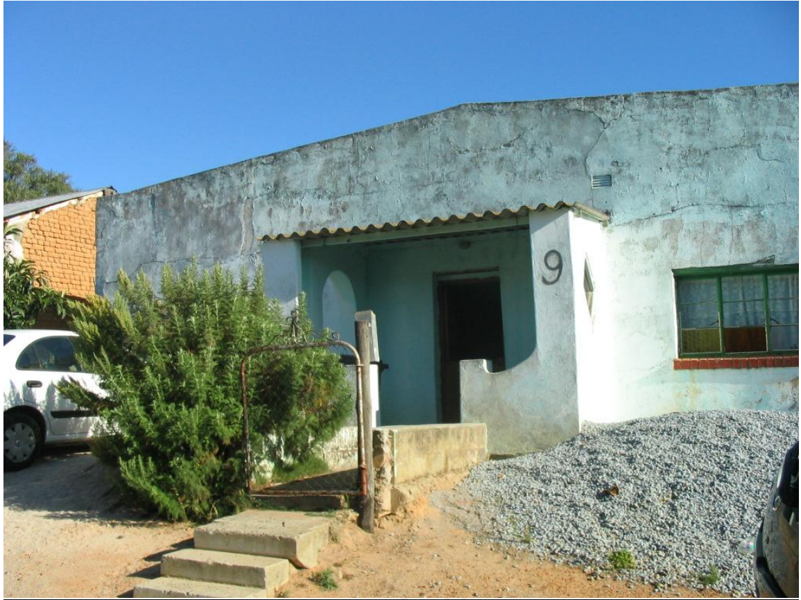
Fig 15: Street façade of dwelling on Erf 326 Mamre
