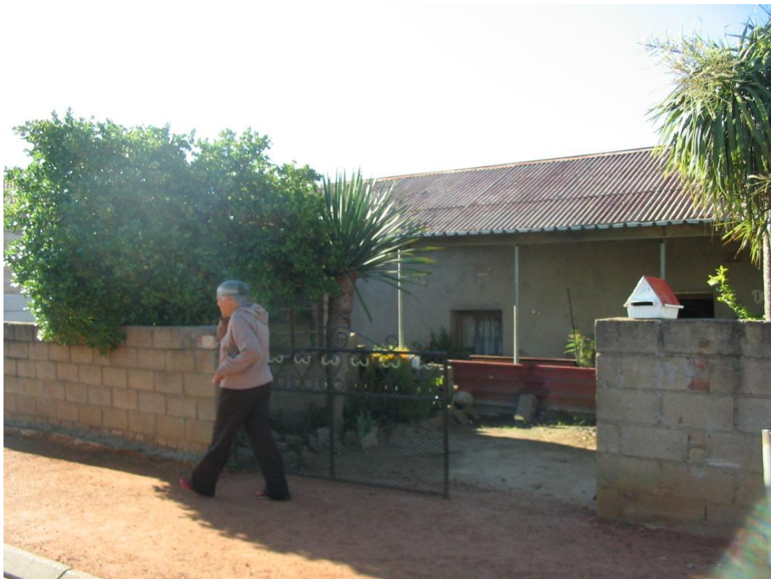
Fig 21: Original rear façade of the dwelling on Erf 285 Mamre; now the entrance,
