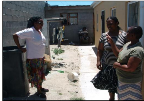
Figure 39b: Concrete aprons sloping towards dwelling; below ground level
