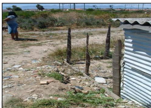
Figure 28d: Planks used to create a barrier to prevent water reaching dwelling (Sweet Home, November, 2010)
