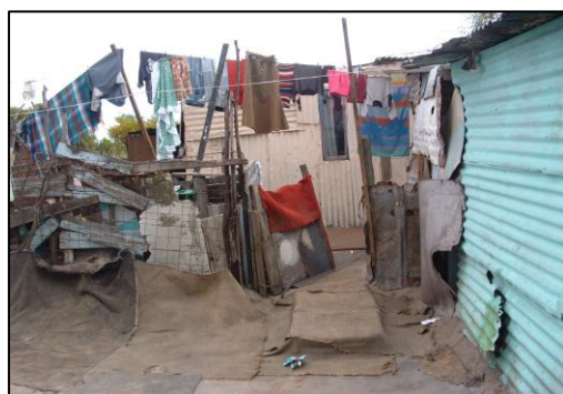
Figure 28c: Raised floor with wooden pallets and carpeting to absorb water (Khayelitsha, June 2006)
