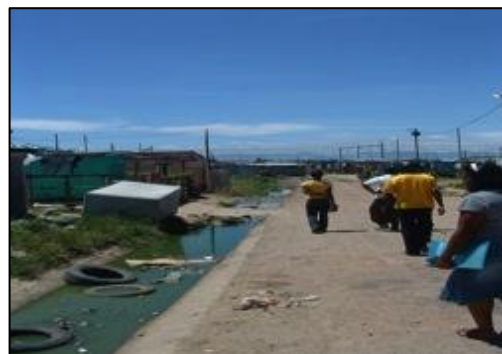
Figure 4d) An illustration of overflowing drainage infrastructure (Sweet Home, November, 2010)
