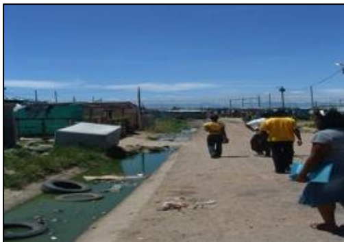
Figure 17: Blocked drainage ditches in Sweet Home informal settlement
