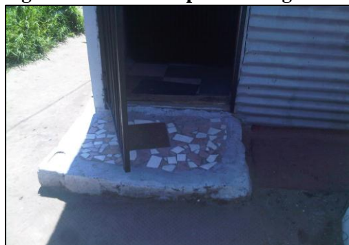
Figure 28a: Concrete floor and step (Kosovo, November, 2010)
